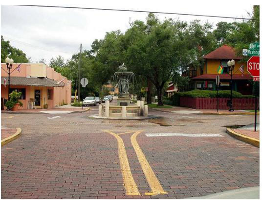
Figure 14 Traffic Circle in commercial setting. Brick pavers, stop signs, and curb extensions serve to slow traffic, reduce pedestrian exposure to vehicles, and maintain visibility. There are no plants on the circle, and no crosswalks. ADA ramps are directly into the path of circulating vehicles, so this may not be an optimal design.
