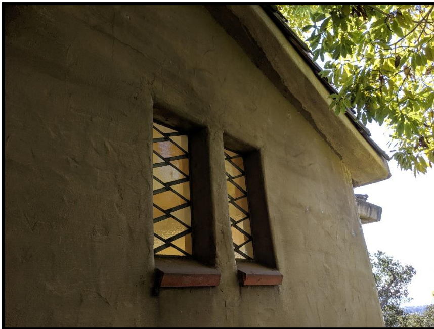
Figure 24:: 4 Mosswood Lane - windows on north facade with leaded design in colored glass
