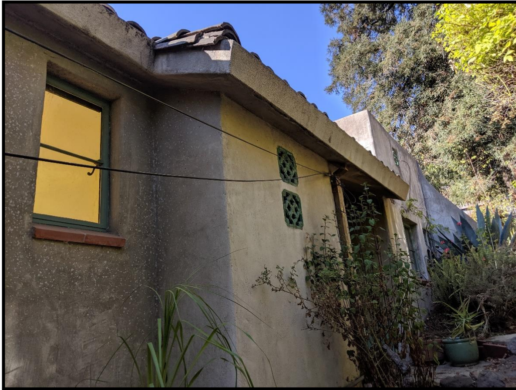
Figure 13: 4 Mosswood Lane - primary (east) façade, facing north
