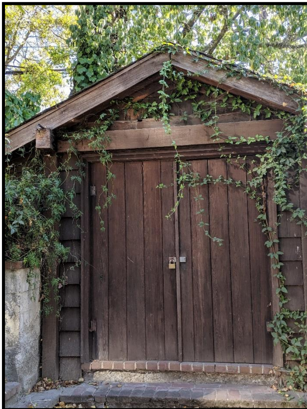
Figure 10: 1 Panoramic Way - accessory structure (playhouse), north façade
