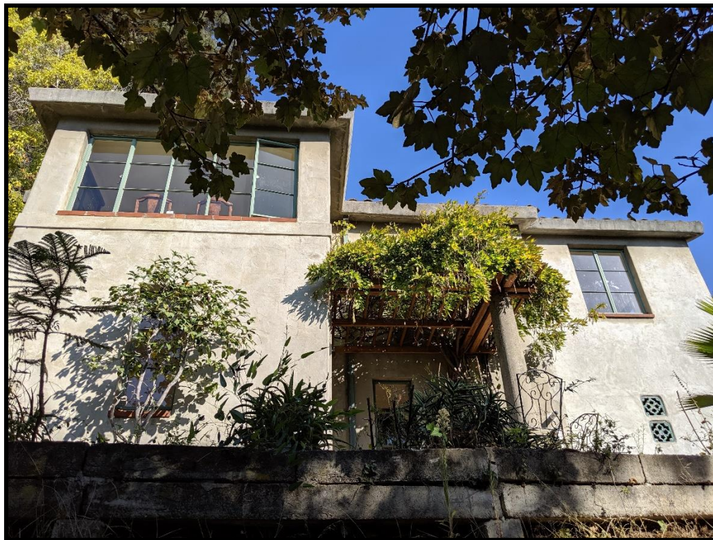
Figure 27: 4 Mosswood Lane - rear (west) facade
