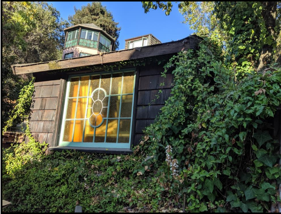
Figure 9: 1 Panoramic Way - accessory structure (playhouse), west façade
