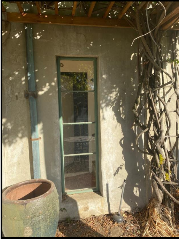
Figure 29: 4 Mosswood Lane - multi-lite window on west façade
