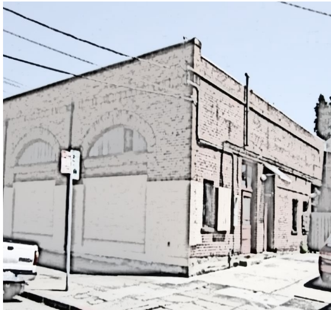
Exhibit 7. Example of unreinforced masonry construction
