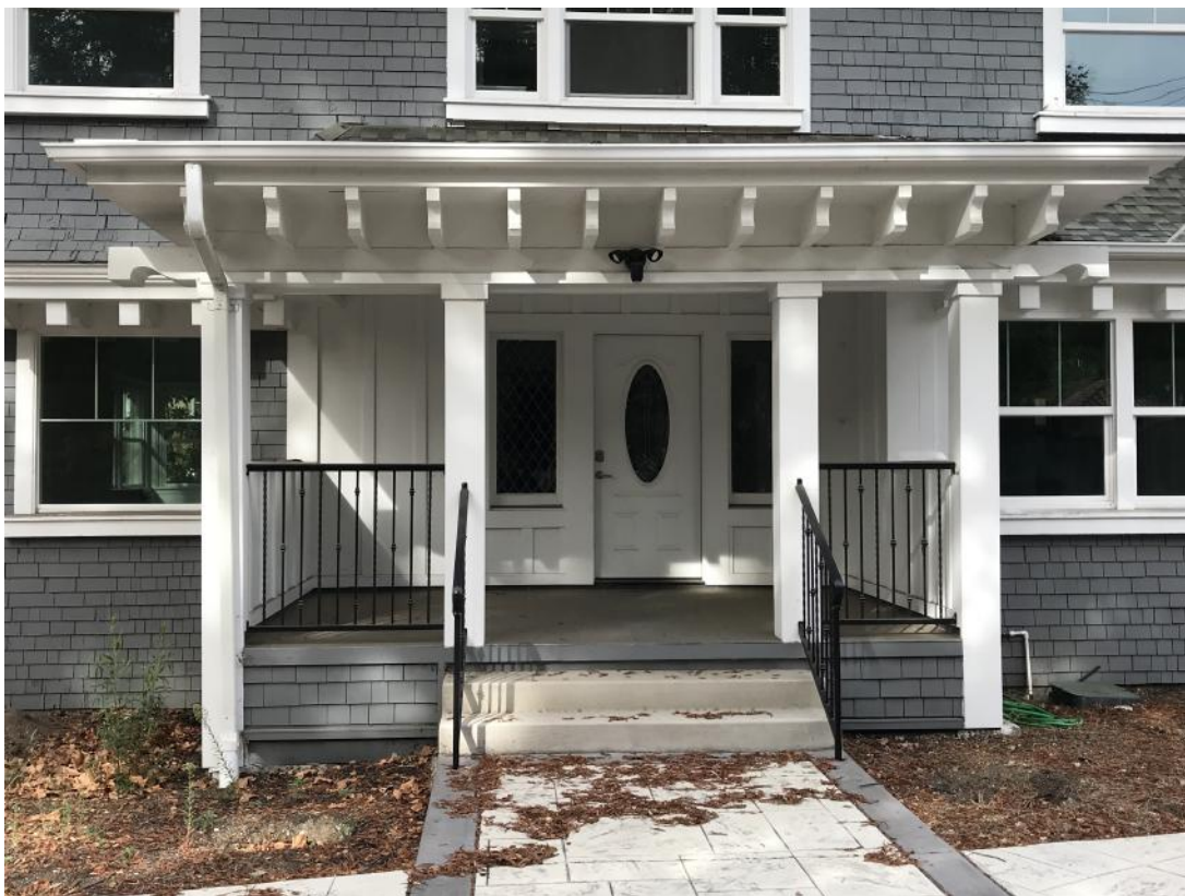
Detail of entry porch, primary (east) facade, looking west.
