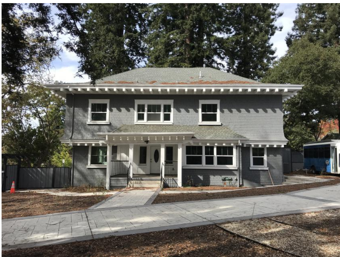
View of primary (east) facade from front of property, looking west.
