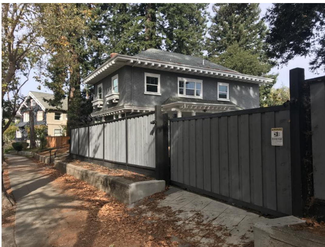
View of south and primary (east) facades from Woolsey Street, looking northwest.
