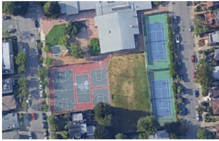
Before: Aerial view of Live Oak – Uneven courts and limited lighting
