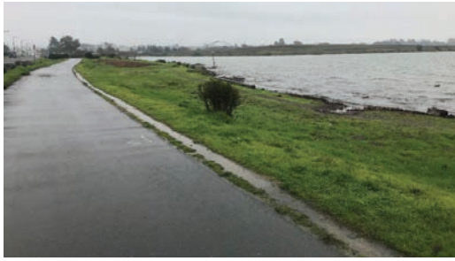
Before: Flood-prone trail
