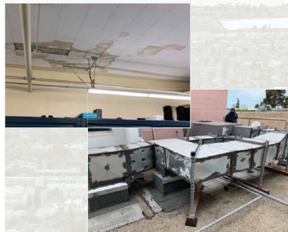
Above Images: Water damage from roof leaks at PSB (top left) and failing HVAC at Fire Station 5 (bottom right).
