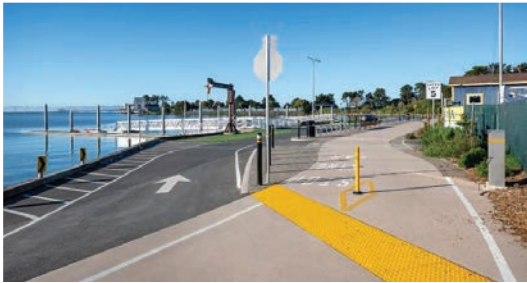
After: Example of Bay Trail Improvements at Berkeley Marina
