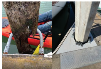
Repair and Improvements to Marina Docks Timber
