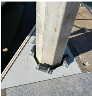
After: New long-life concrete piles
