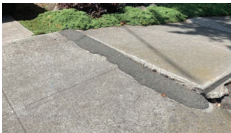
Before: Damaged sidewalks and long repair waitlist
