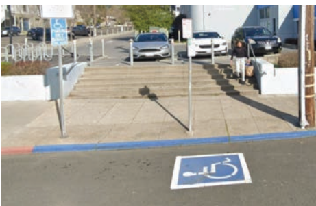
Before: On-street accessible parking with blocked sidewalk access, creating barriers for wheelchair users and pedestrians.
