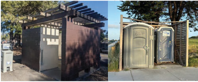
Before: Example of open cinderblock restroom at Codornices Park (left) and temporary restrooms at Cesar Chavez Park (right)
