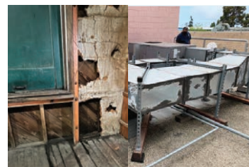
Repair and Improvements to Public Safety Facilities
