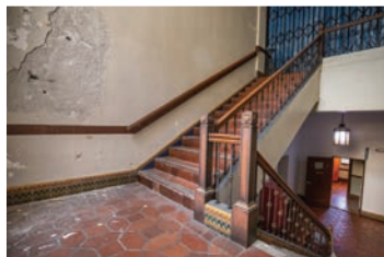
Repair and Improvements to Veterans Building
