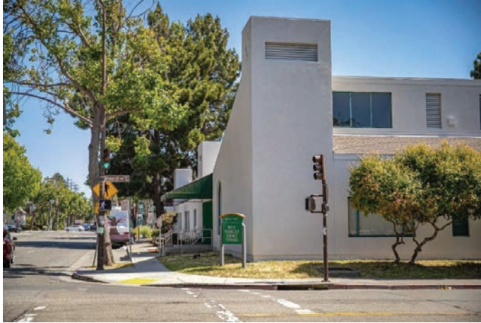
Before: Current exterior of West Berkeley Family Wellness Center
