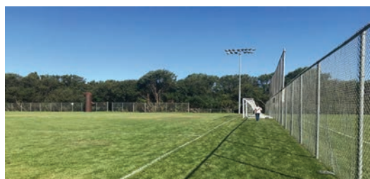
Before: Existing field conditions
