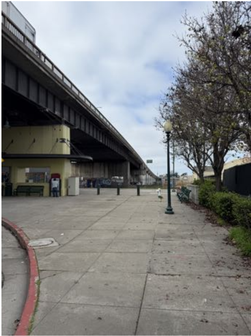
VIEW ALONG UNIVERSITY AVE. TOWARDS WEST
