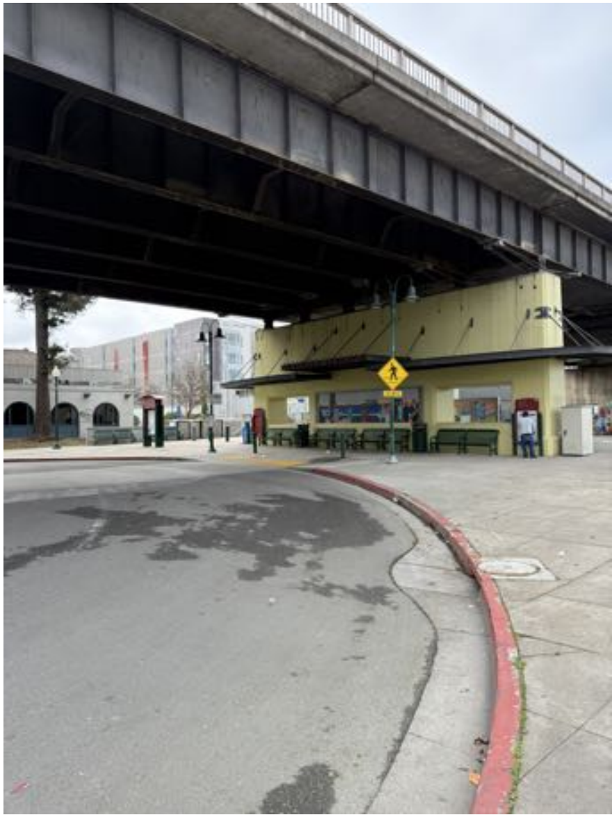
VIEW ALONG UNIVERSITY AVE. TOWARDS WEST
