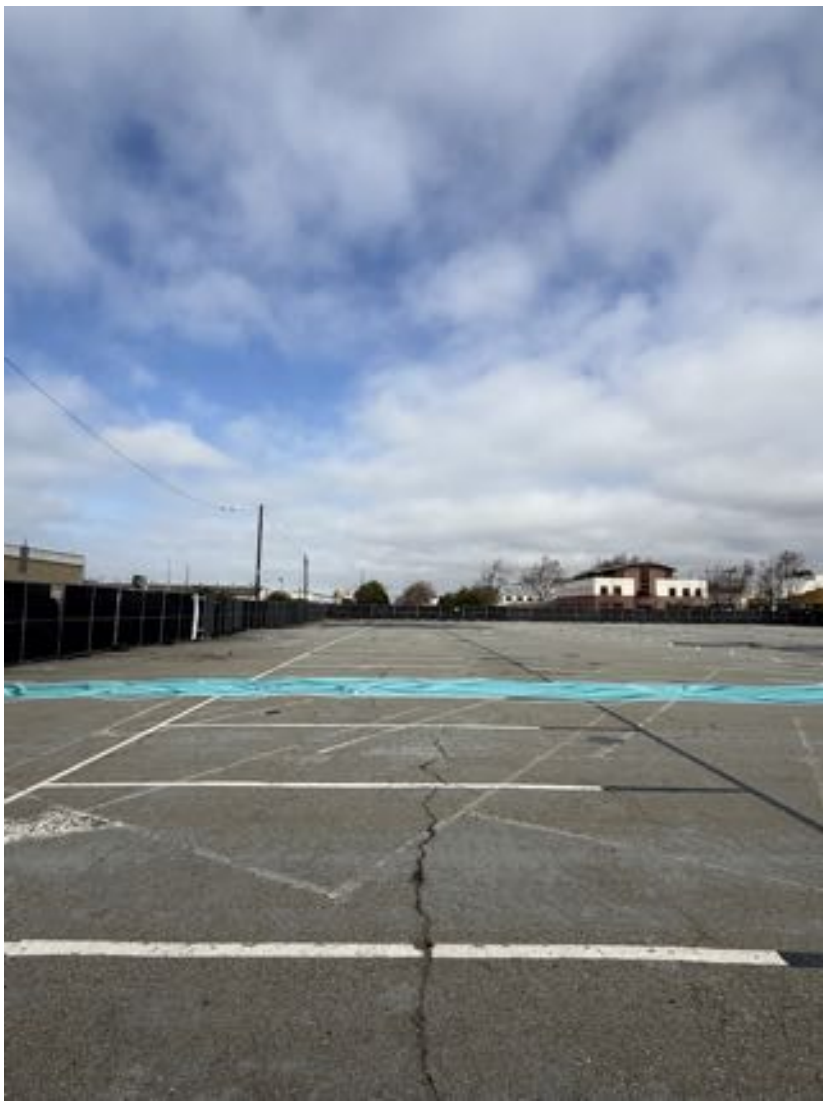
EXISTING PARKING LOT IN SUBJET PROPERTY
