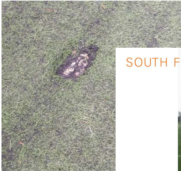
CARPET DAMAGE AND SPOT REPAIRS
