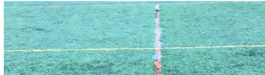
CARPET DAMAGE AND SPOT REPAIRS
