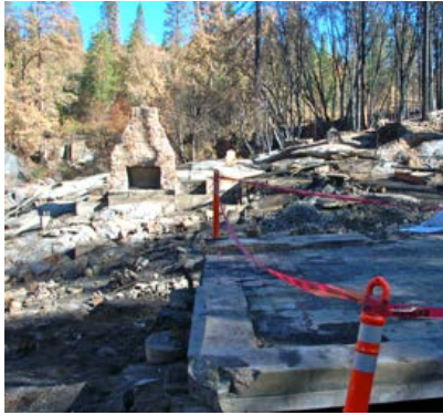
Dining Hall after fire (10/30/13)
