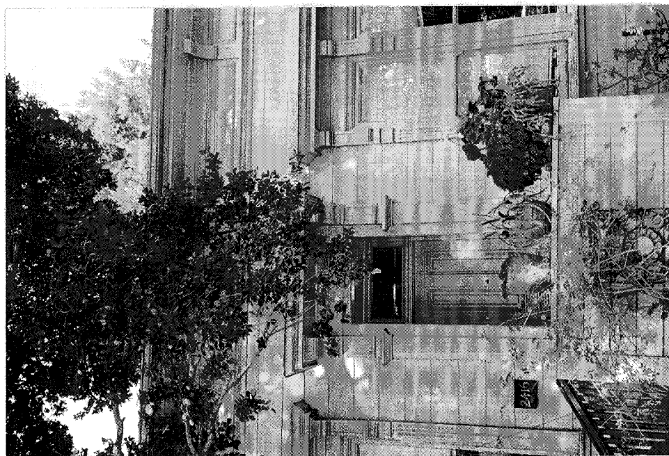
Figure 3. Front entrance, and adjacent window, with cornices and sidepieces
