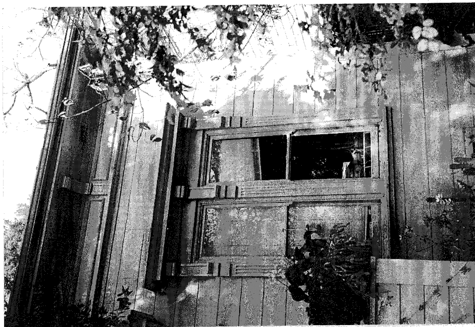
Figure 4. Living-room windows and their surrounds
