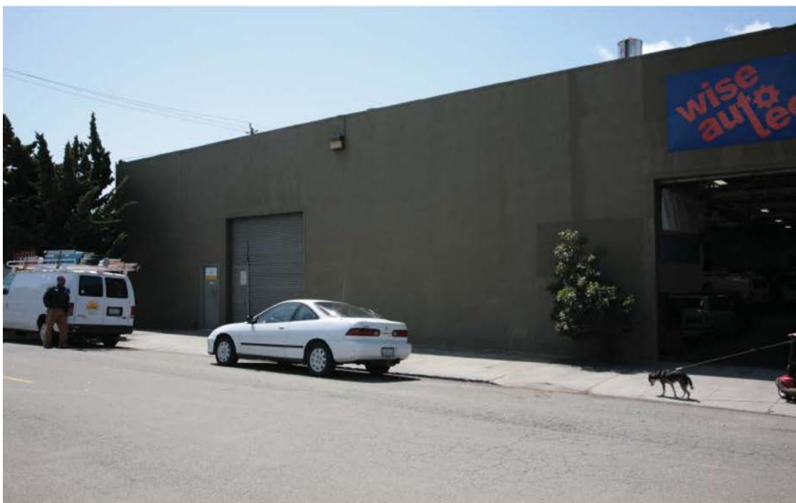
Photo 2: 2710 Tenth Street, looking southwest. (Shayne Watson, 2018)
