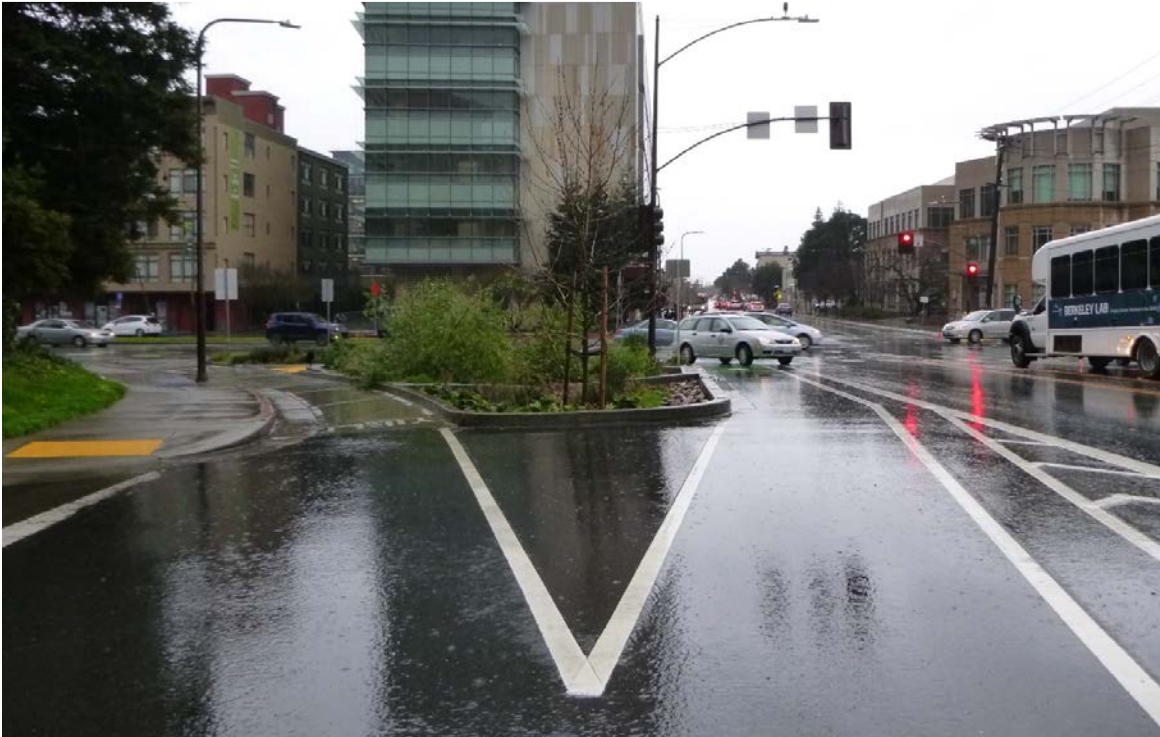
Figure 6 – A bioretention facility was installed along with pedestrian and cyclist safety improvements as part of the Hearst Complete Streets Project.
