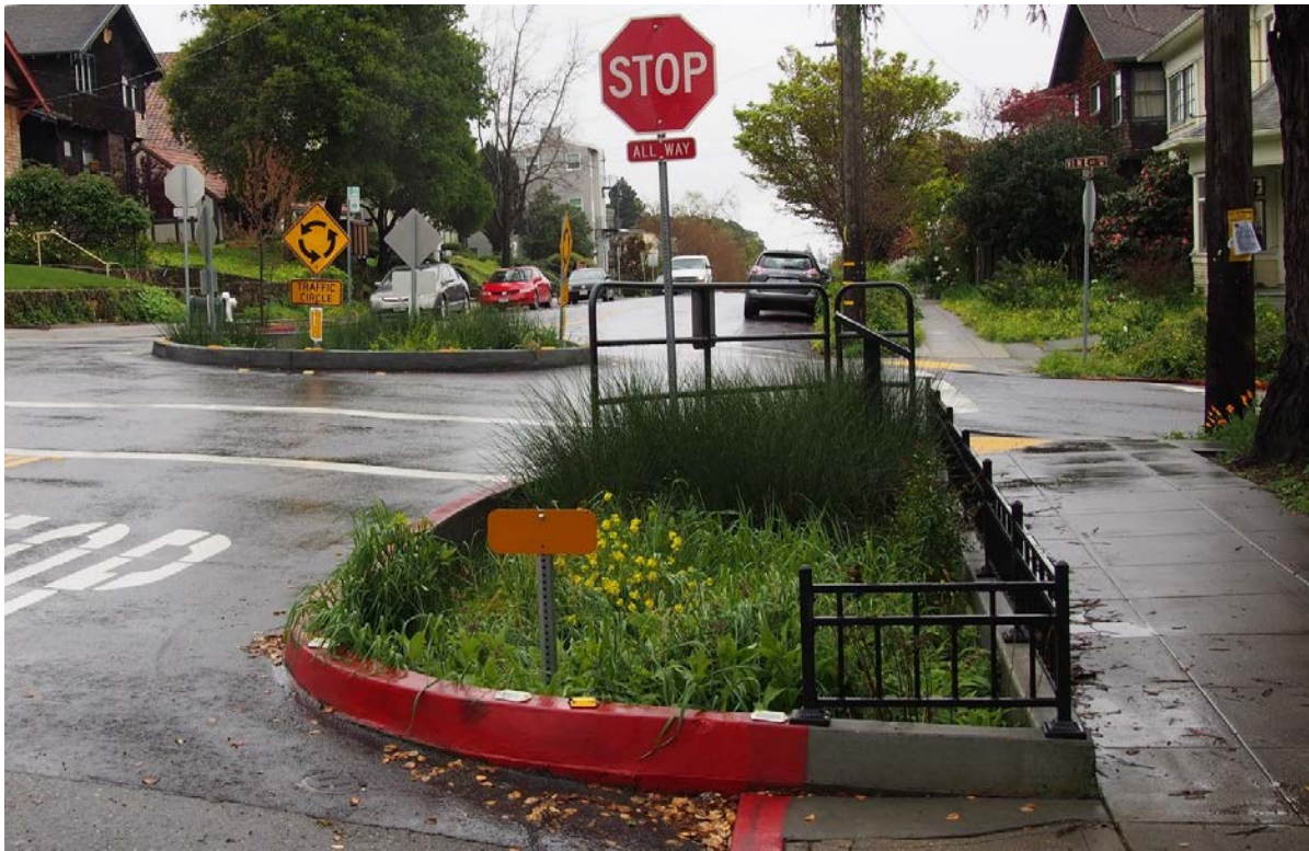
Figure 7 – Connected bioretention features in a traffic circle and corner bulb-out at Spruce and Vine Streets.
