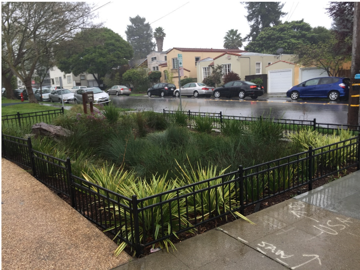
Figure 19 – An existing bioswale at Presentation Park detains, treats, and infiltrates runoff from Allston Way.
