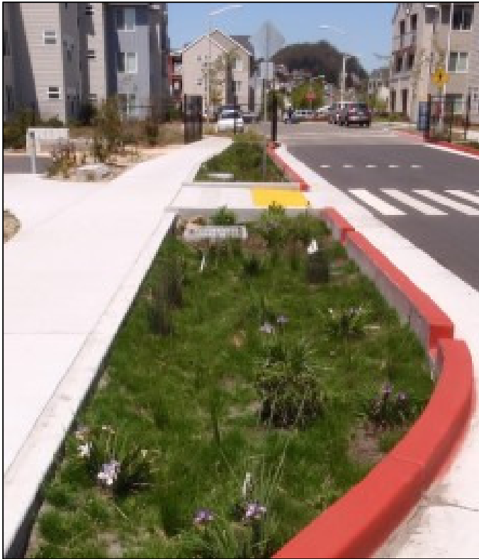
Figure C-9. Curb Extension. In addition to reducing the street width and shortening the length of street crossings for pedestrians, curb extensions, or “bulbouts,” such as this example in Albany, also provide space for GI facilities.
