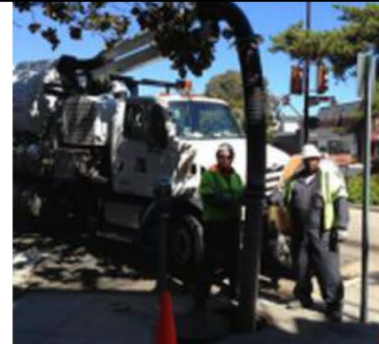
Public Works Crew Cleaning Sewer Lines
