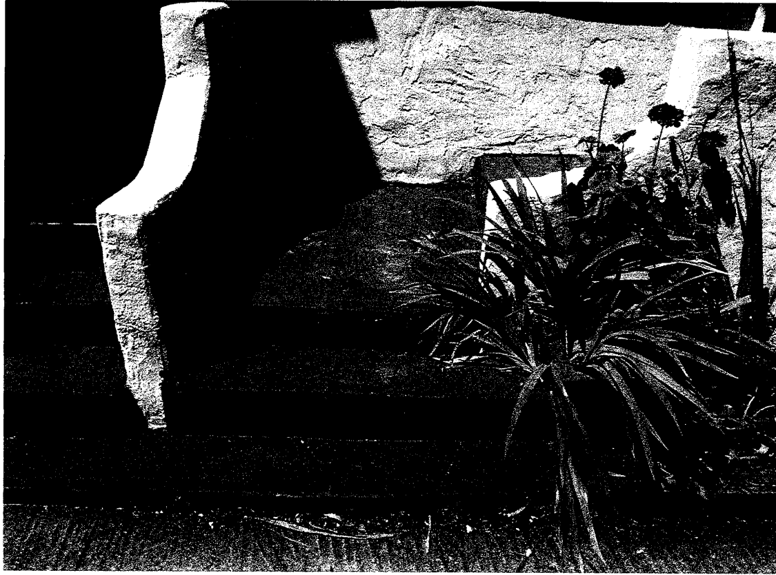
Apt F steps and apartment entranceway barriers
