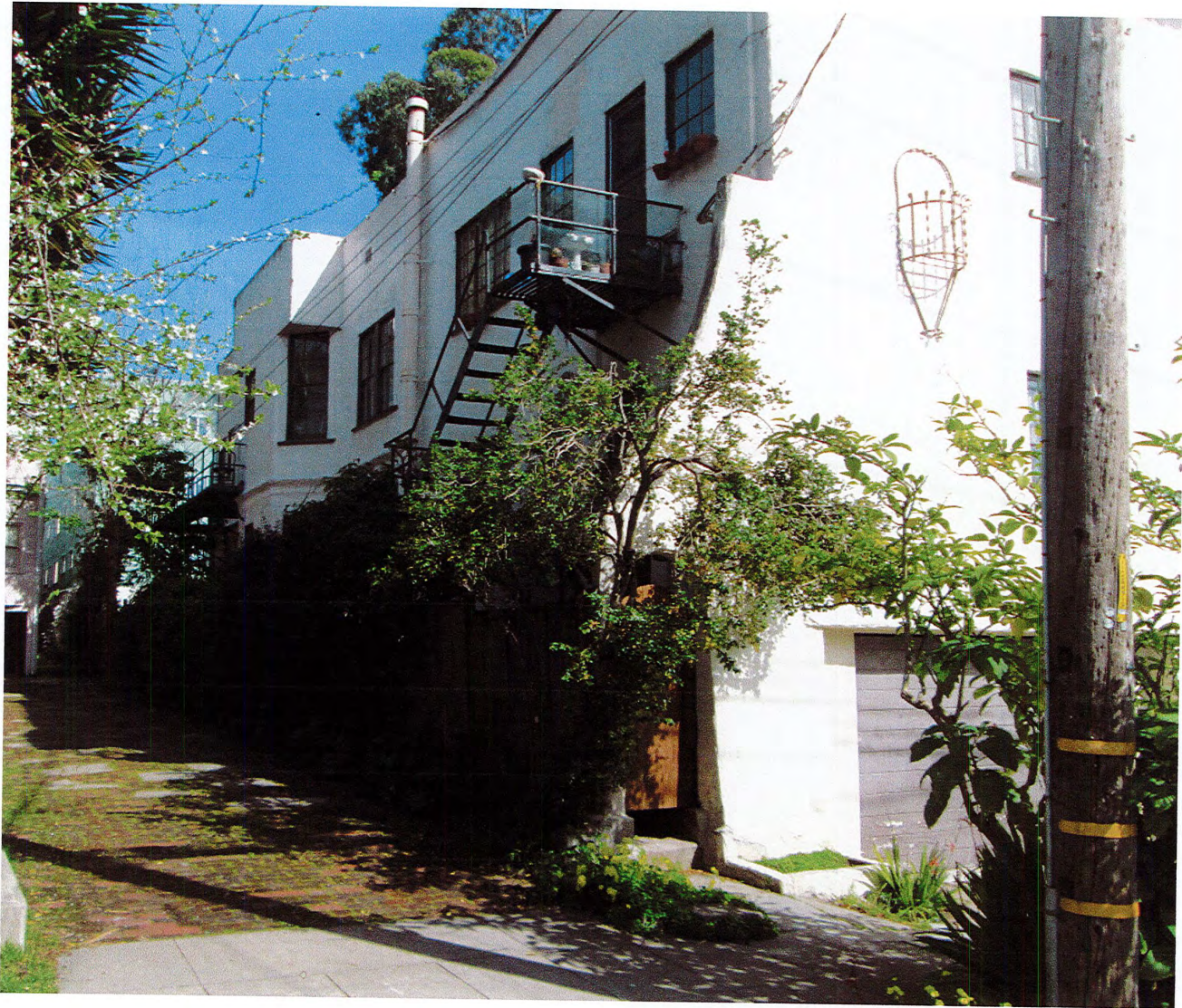
North side of 1619 Walnut (photo is facing east)
