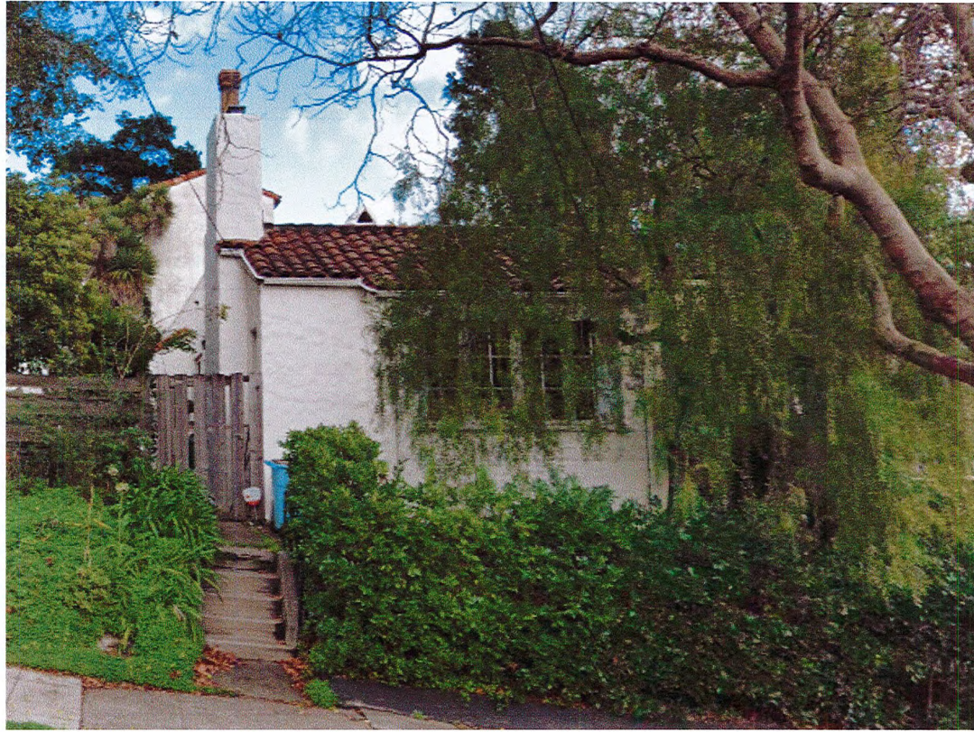
1611 Euclid (1924 William Alexander Doctor) – Builder: Evan D. Bramlage - Owner: Mabel M. Bramlage
