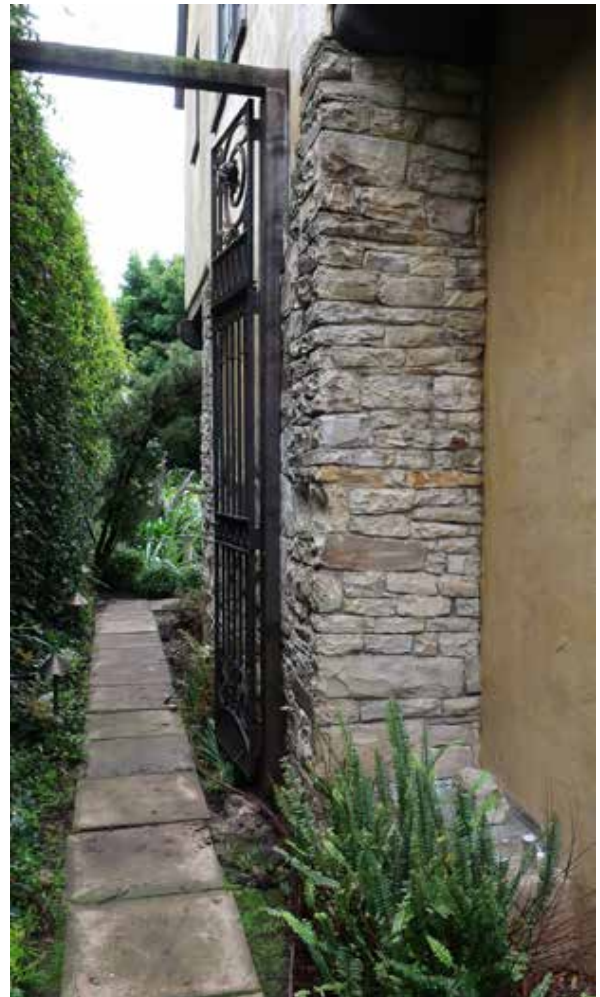
Fig.55 - Rear path at east-facing gable
