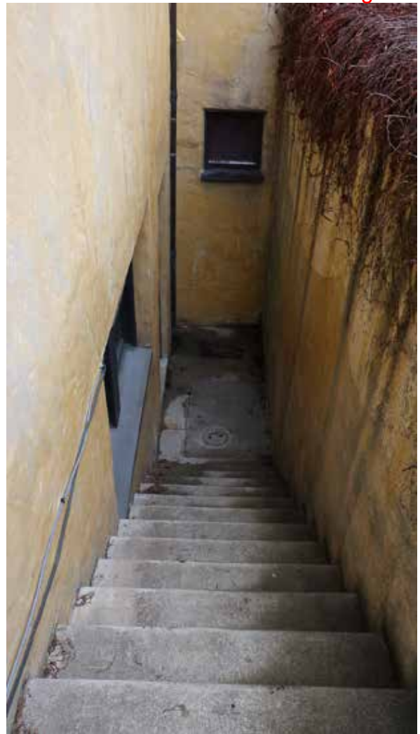
Fig.36 - Basement stair at north side
