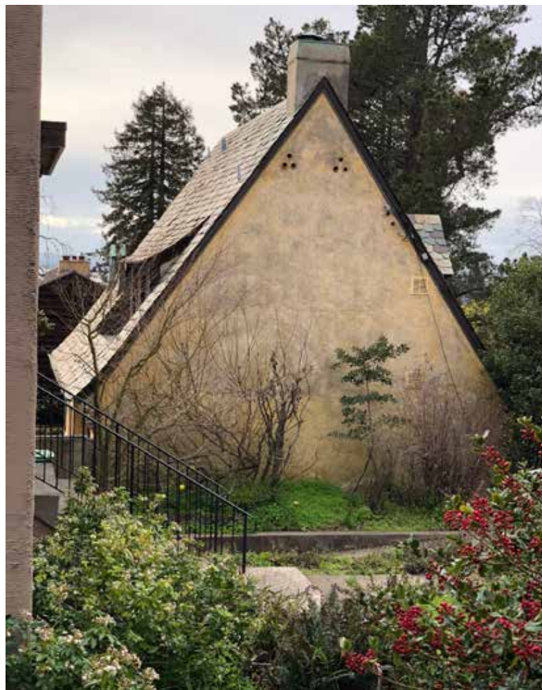
Fig.51 - Carriage house east side
