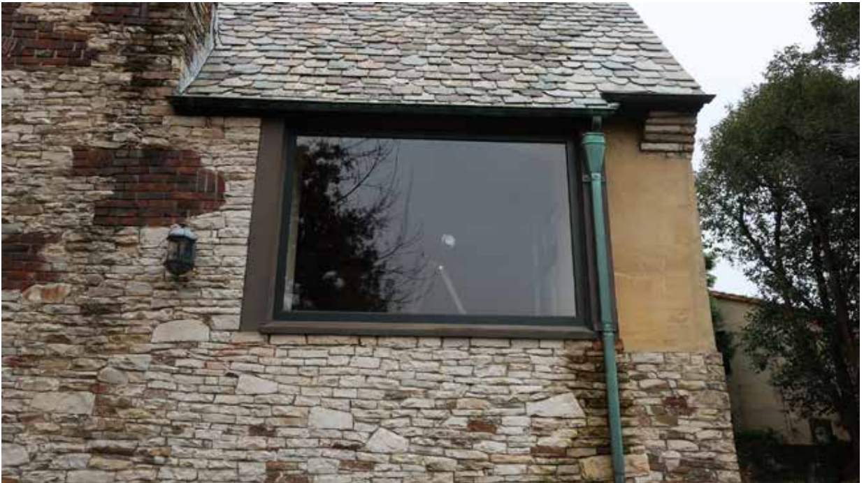
Fig.27 - Picture window at south end of front facade
