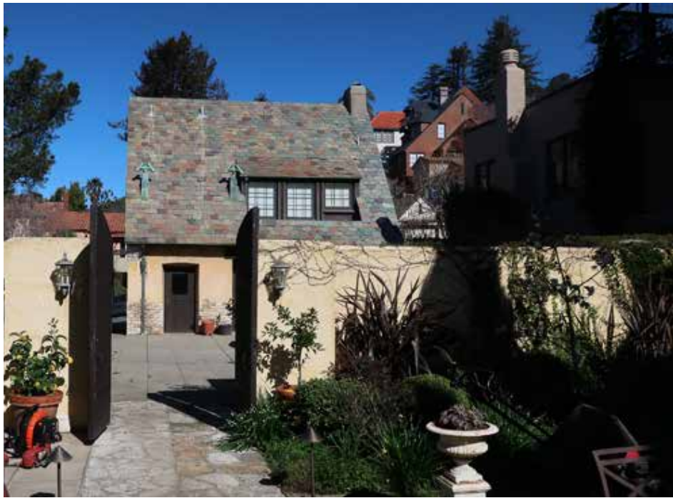
Fig.47 - Carriage house rear from rear yard
