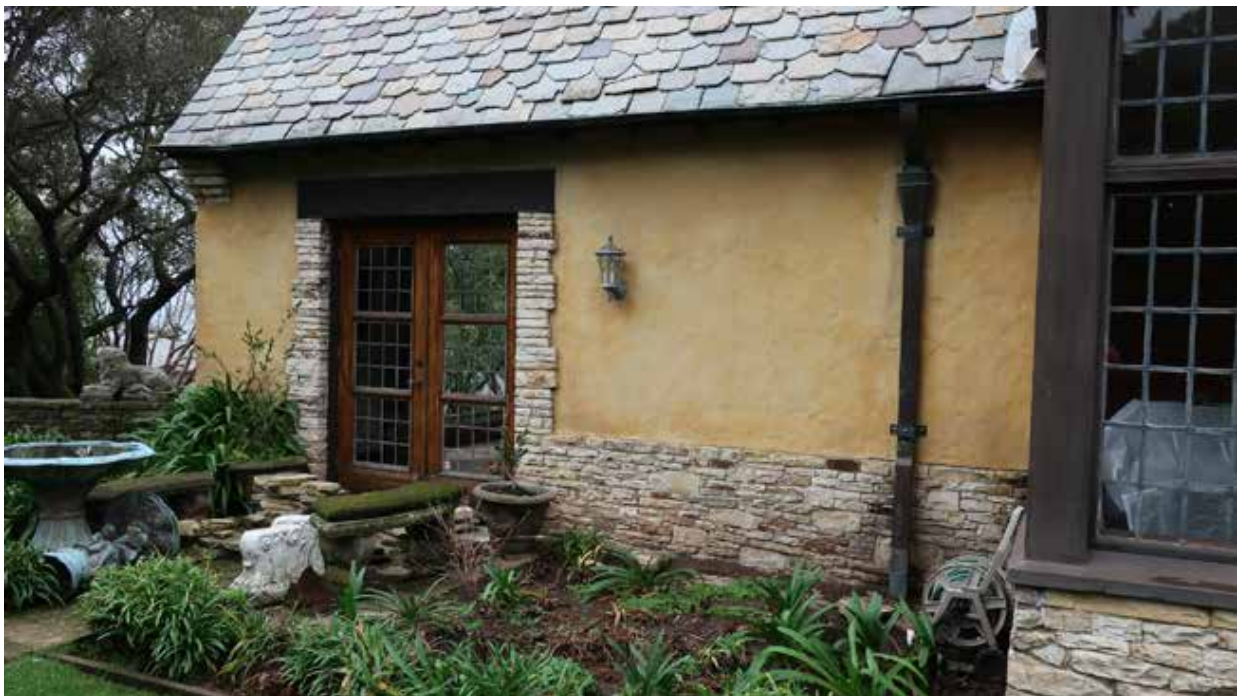
Fig.46 - South end rear elevation
