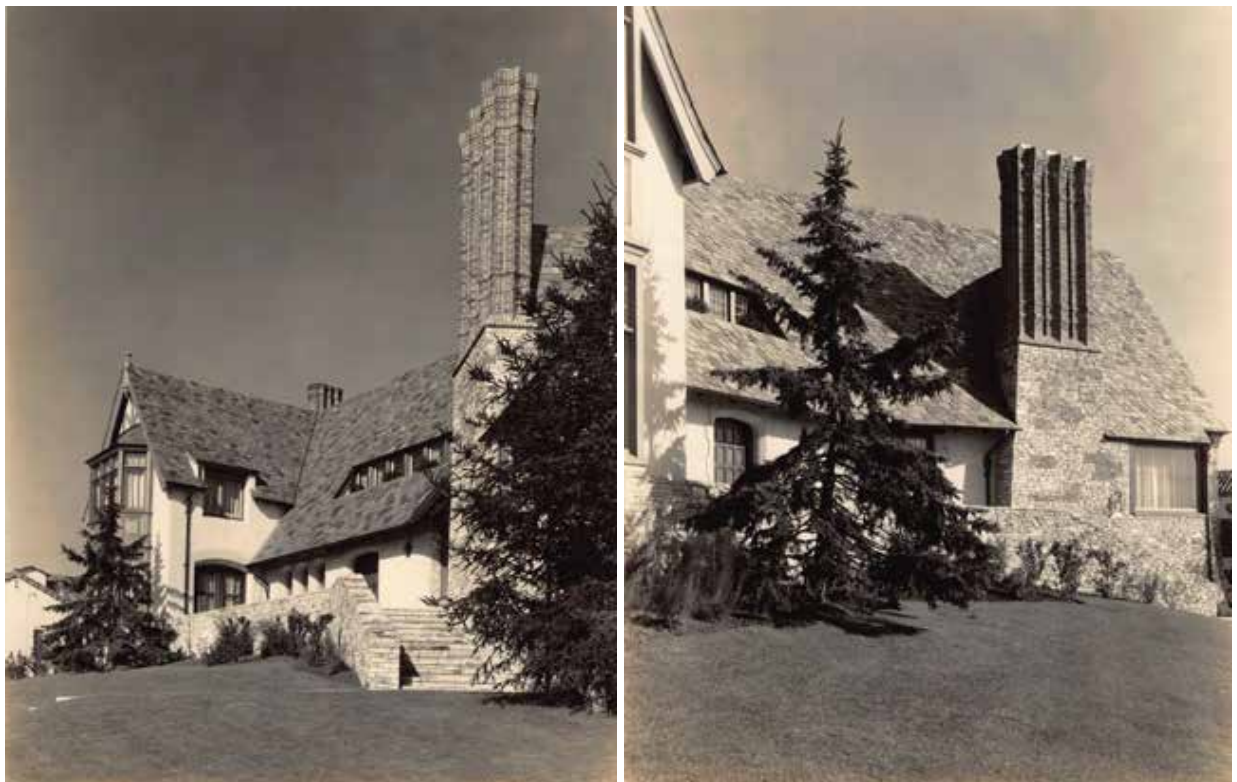
Figs.11-12 – Front views, 1931, looking northwest (at left) and northeast (courtesy Ratcliff)
