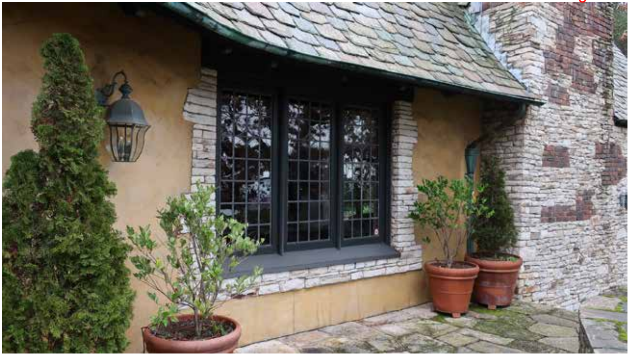
Fig.23 - Front windows at right (south) side of entry door
