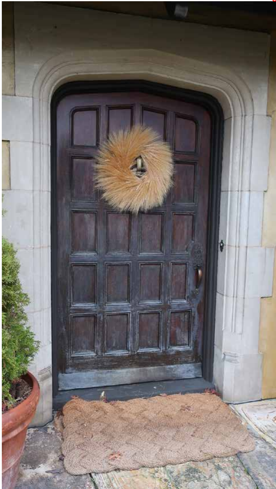
Fig.22 - Front entry door
