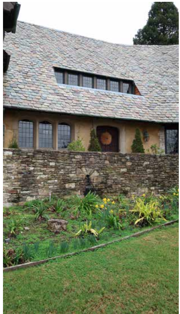
Fig.18 - Front terrace, entry way and roof
