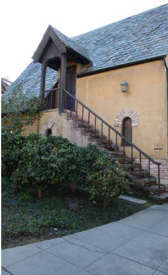
Fig.48 - Carriage house front (north)
