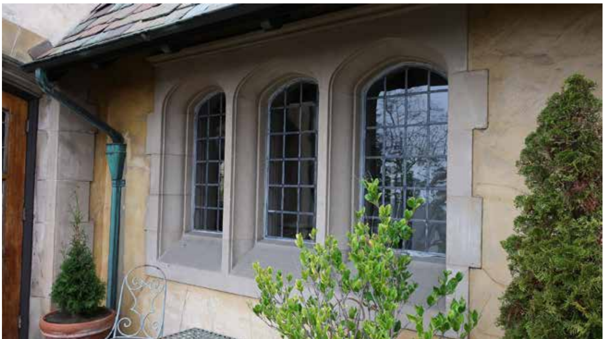
Fig.24 - Front windows at left (north) side of entry door
