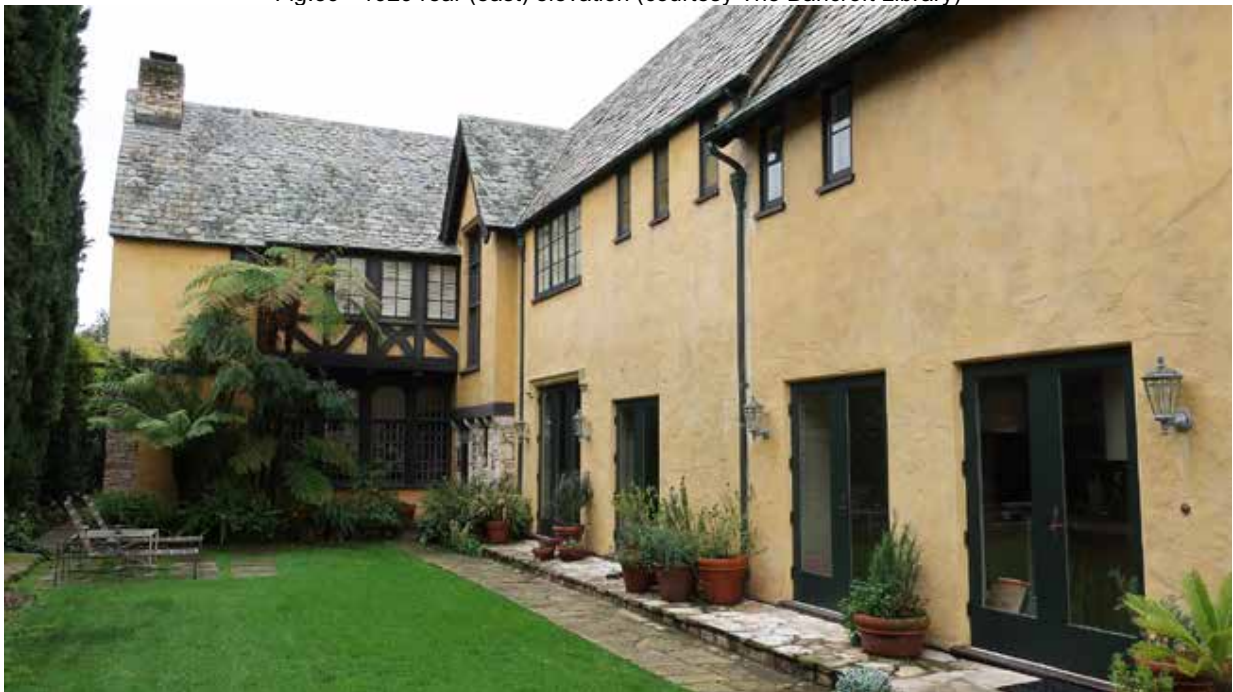
Fig.40 – Rear (northern side)
