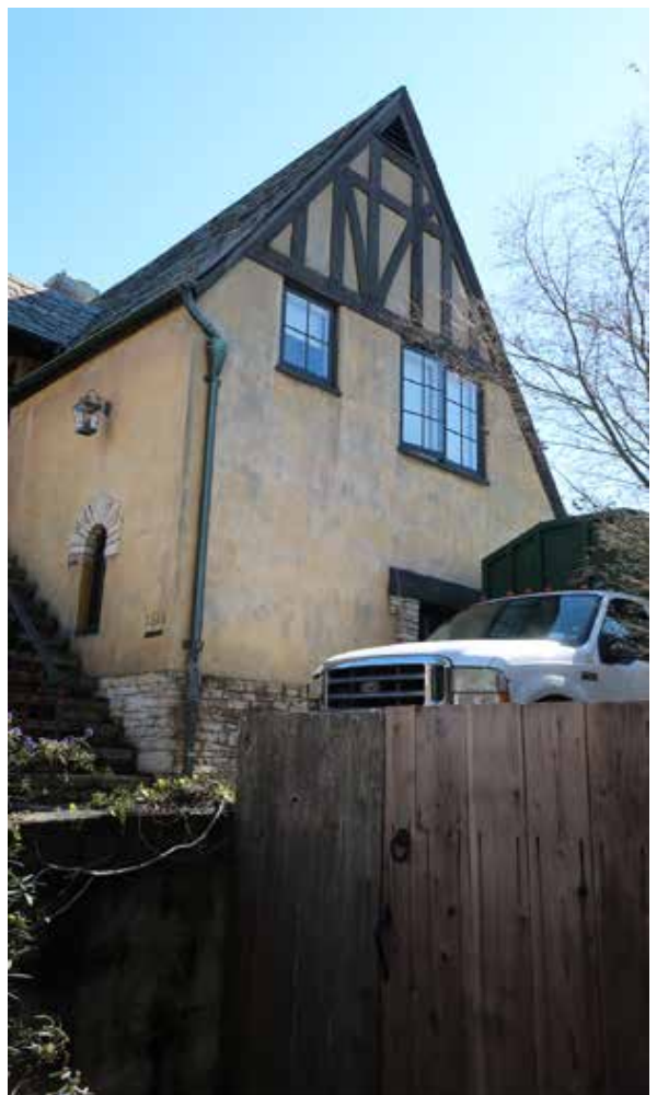
Fig.49 - Carriage house west side
