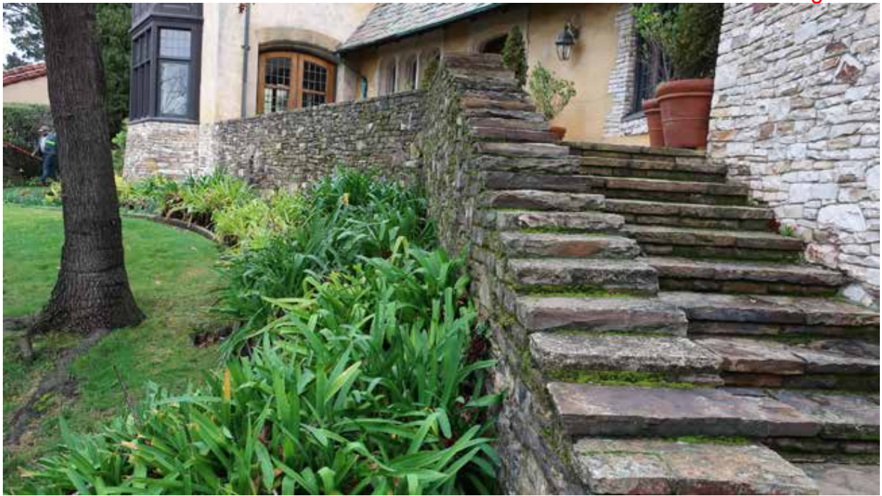
Fig.19 - Front terrace and entry steps
