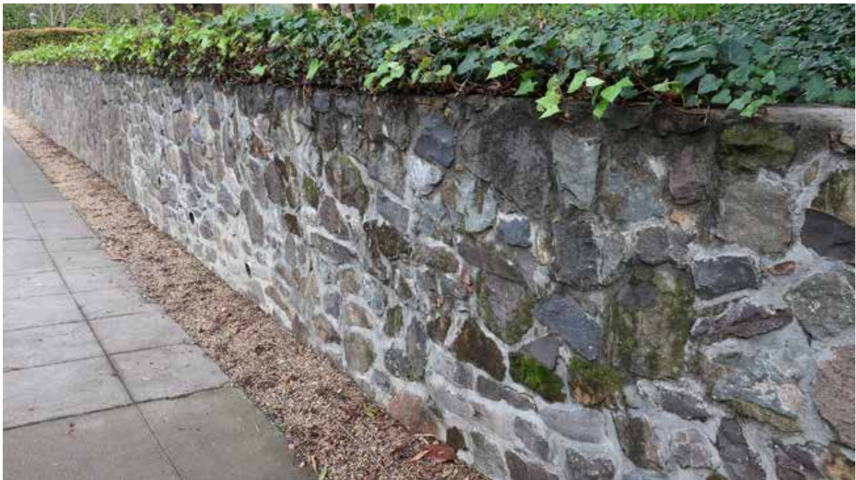
Fig.52 - Site wall at Euclid Ave. sidewalk
