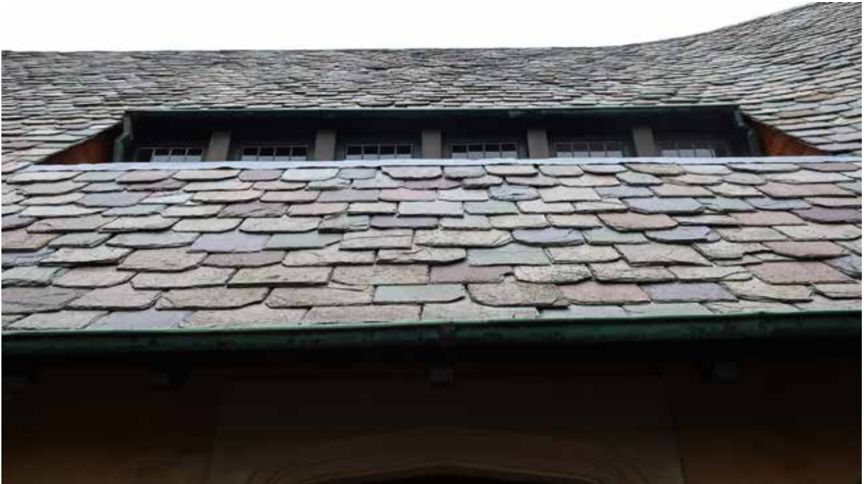
Fig.26 - Window opening at front roof
