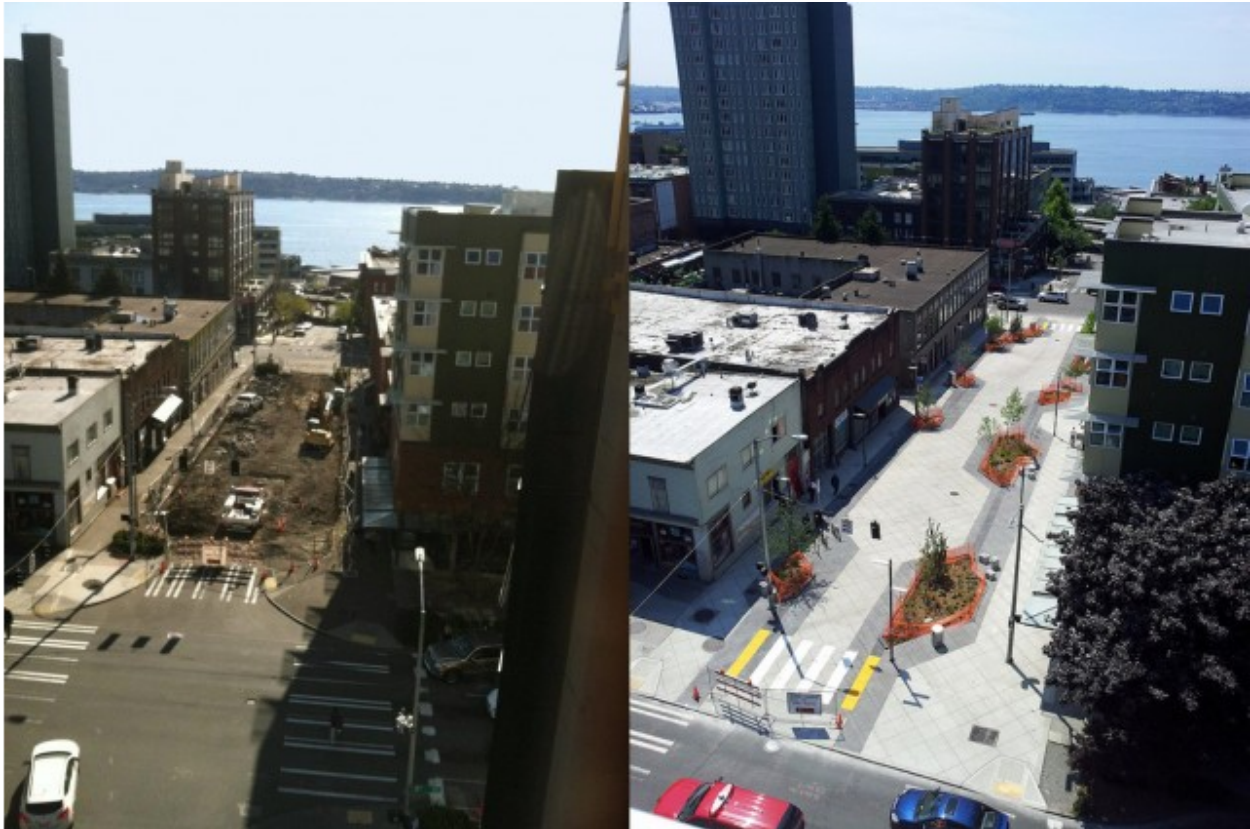
Bell Street, during and shortly after construction.
