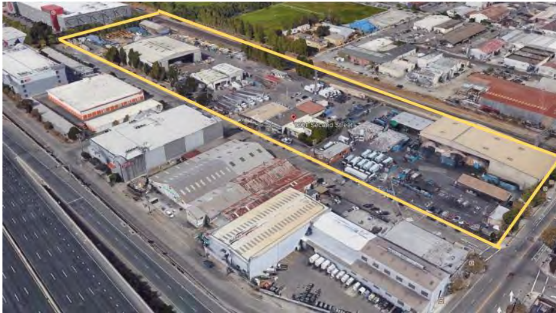
Figure ES-2: Aerial Overview of Existing Recycling and Solid Waste Operations on 2 nd St.
