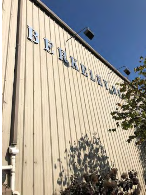
Figure 37: Facility ID Signage on South wall of MRF building
