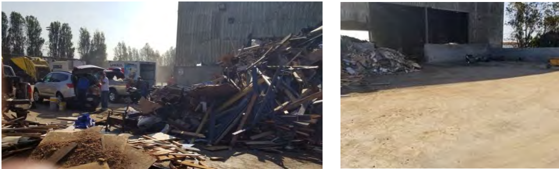
Figure 8 & 9: Public Tipping Area North Side C&D Outdoor Drop-Off Area
