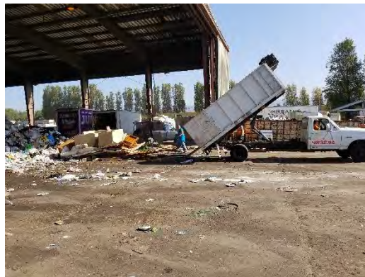
Figure 18: South Side View of Transfer Station
