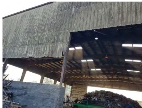
Figure 10: North Side View of Transfer Station
