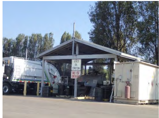
Figure 12: Used Oil Canopy
