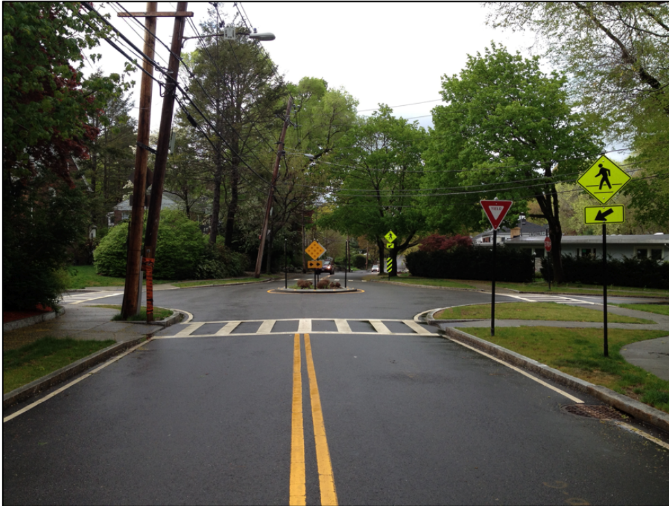
Figure 21 Image of a neighborhood traffic circle in the NACTO Urban Street Design Guide featuring low ground cover and no trees. This image was also used in Reference 1.
