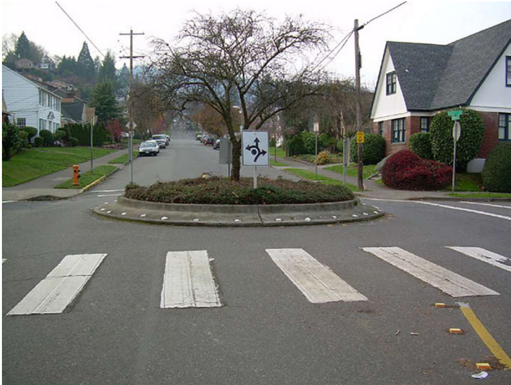
Figure 16 Potential Pedestrian-Vehicle conflict at traffic circle because the circle is too close to the crosswalk
