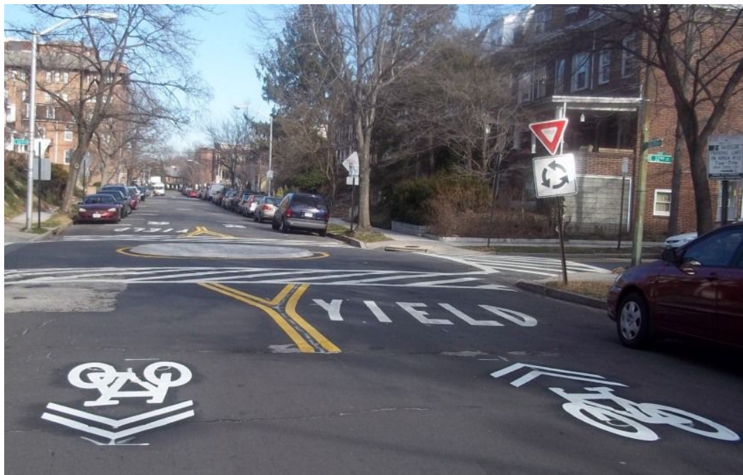
Figure 28 A fully mountable traffic circle in Baltimore, MD, with no signs or planting in the intersection.
