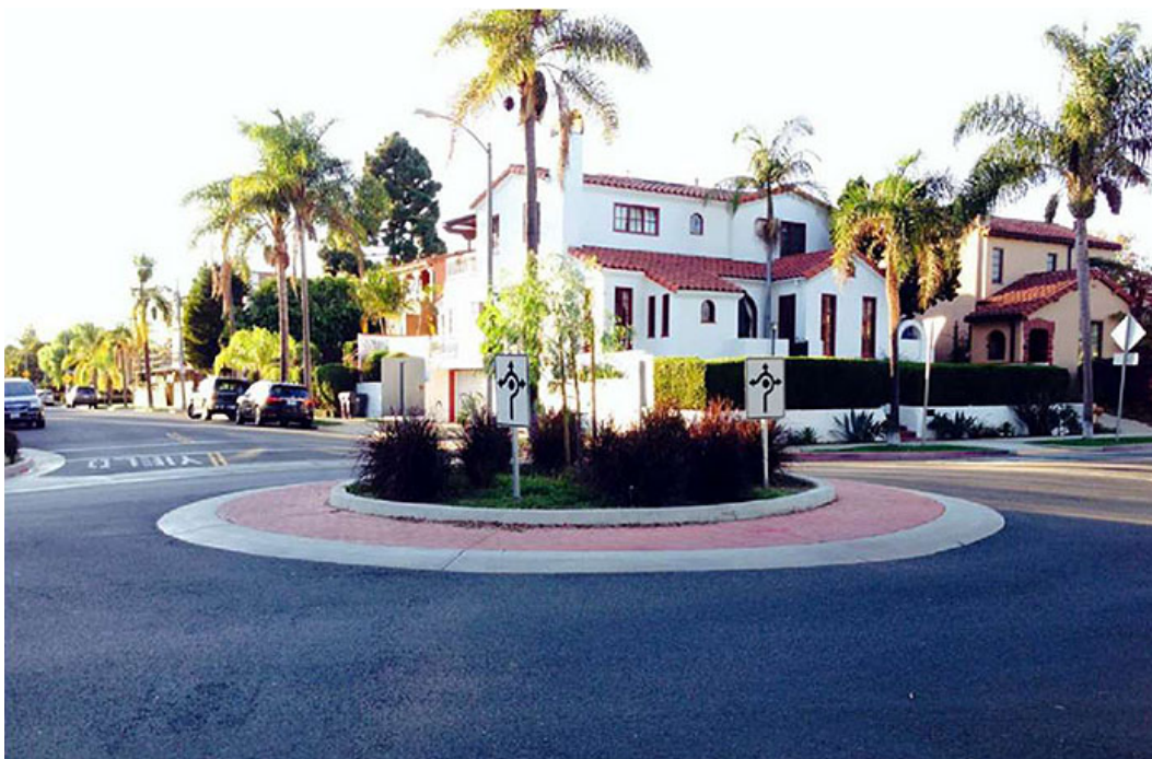
Figure 15 Traffic circle in residential setting, with wide mountable curb, guide signs, yield control on approaches
