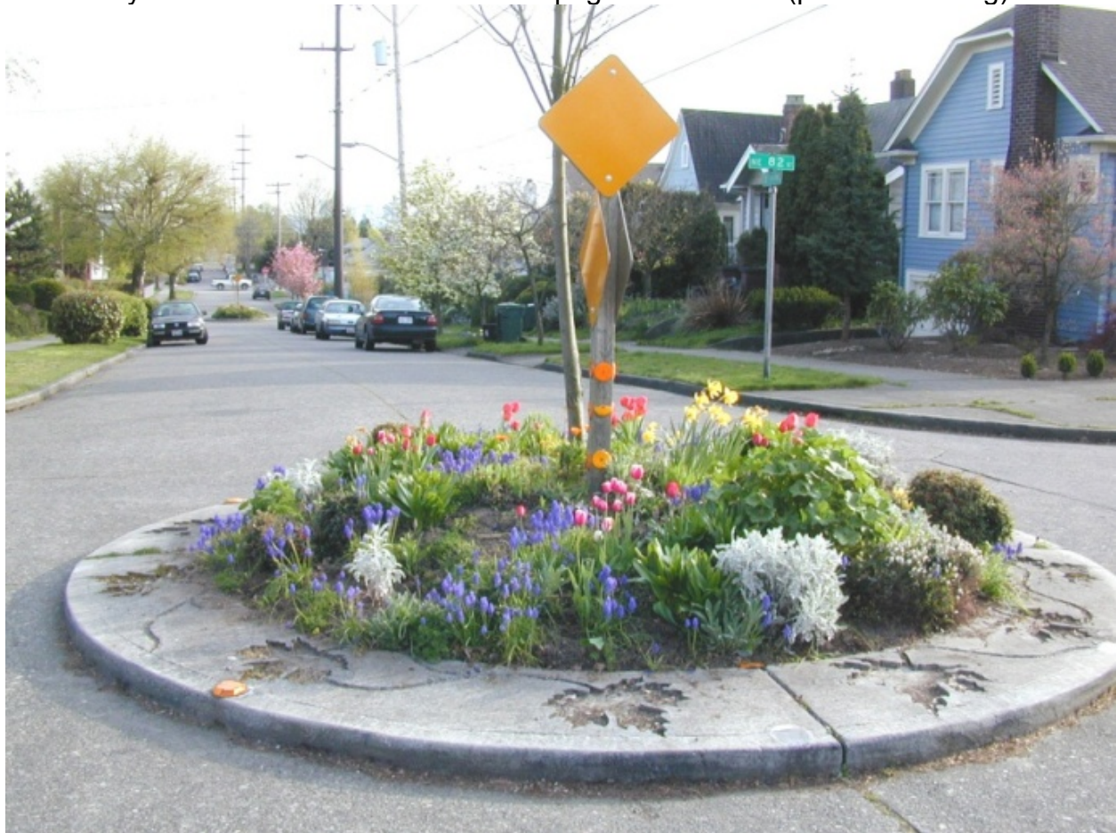
Figure 8 This traffic circle in a Seattle neighborhood also incorporates stamped concrete.
