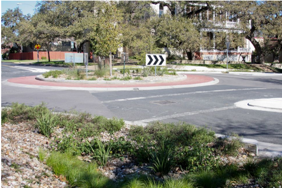
Figure 27 This is more of a roundabout than a neighborhood traffic circle. It features a mountable apron, directional signs, low ground cover, and a small tree.
