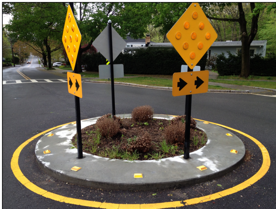
Figure 20 Image of a neighborhood traffic circle in the NACTO Urban Street Design Guide featuring low ground cover and no trees. This image was also used in Reference 1.
