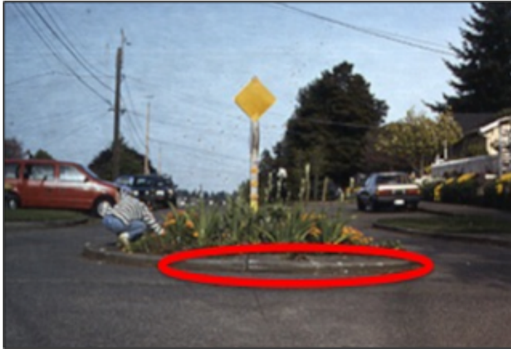
Figure 6 Traffic Circle with Scraped Curb from Heavy Vehicle Traffic
