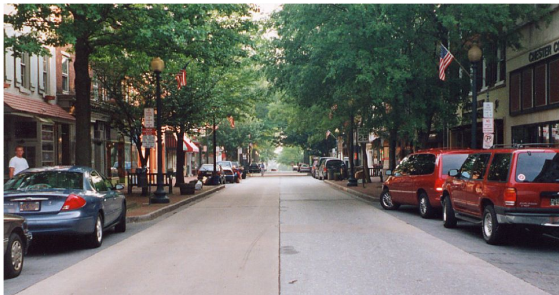
Figure 30 Commercial street with midblock curb extensions featuring trees
