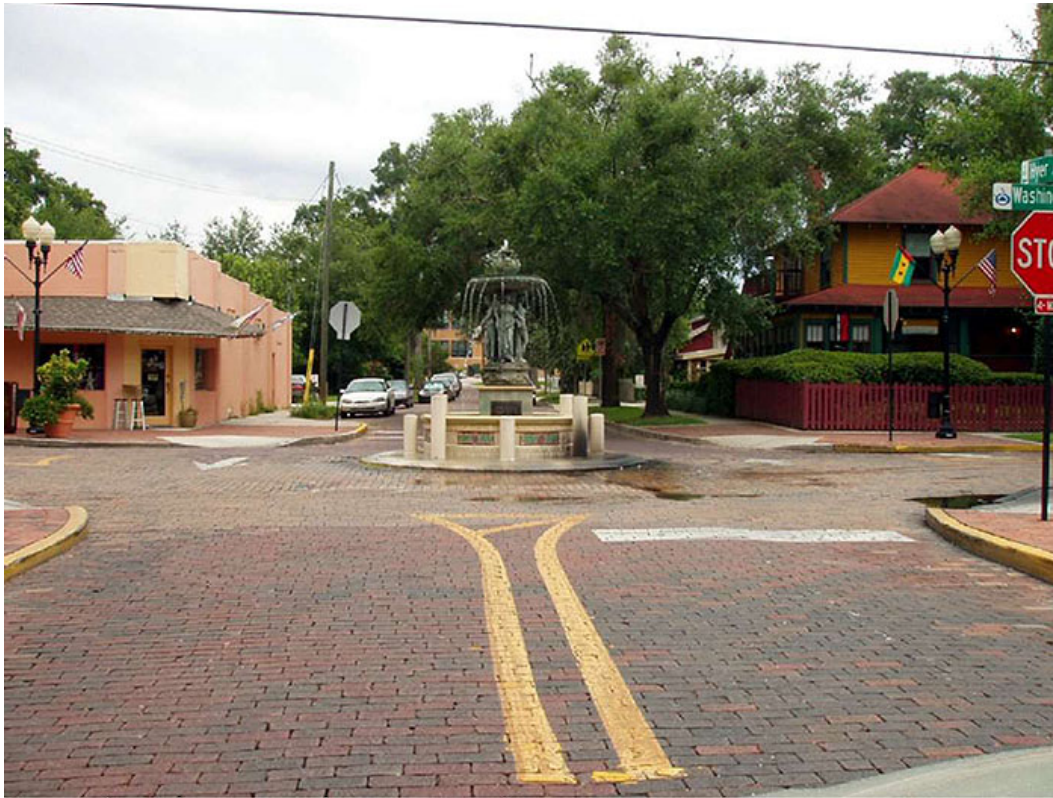
Figure 14 Traffic Circle in commercial setting. Brick pavers, stop signs, and curb extensions serve to slow traffic, reduce pedestrian exposure to vehicles, and maintain visibility. There are no plants on the circle, and no crosswalks. ADA ramps are directly into the path of circulating vehicles, so this may not be an optimal design.
