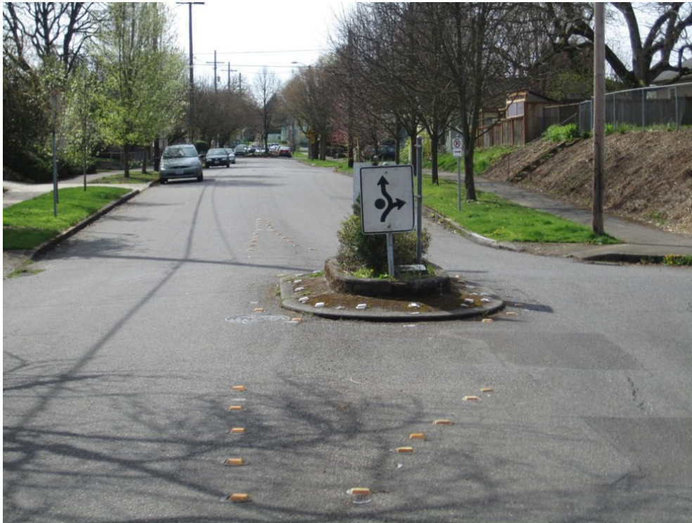
Figure 25 Image of a neighborhood traffic circle in the NACTO Urban Street Design Guide featuring an oval shape, low ground cover, and no trees.
