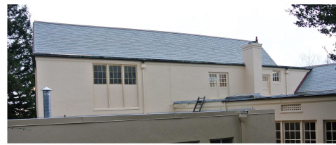
NORTH ELEVATION PHOTO
