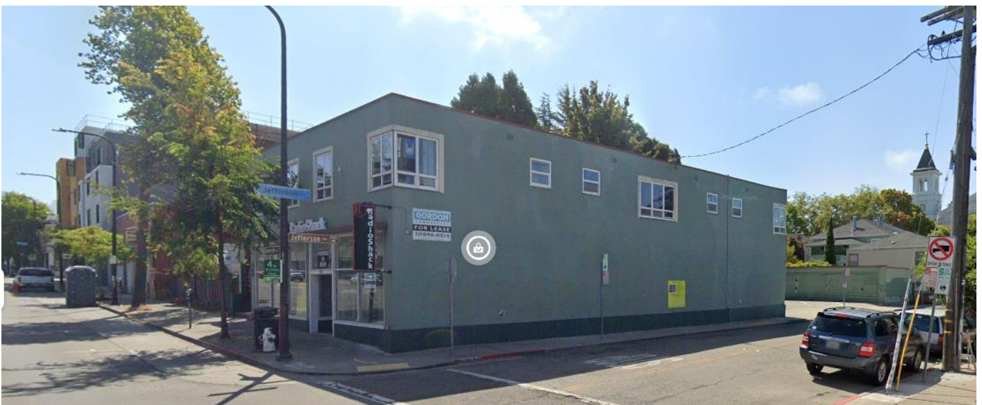
Figure 3: 1652-1658 University Avenue – Current site conditions, northwest elevation (Google; 2022)
