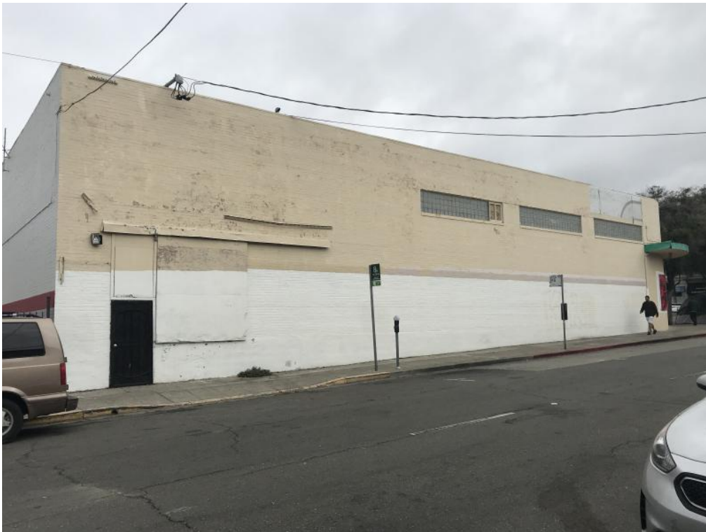
South facade, looking northeast from Haste Street.
