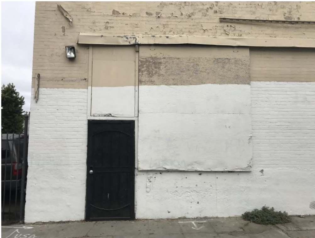
Detail of service entrance, south facade.
