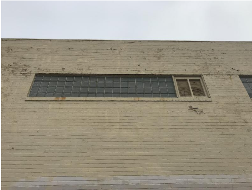
Detail of glass block window, upper south facade.
