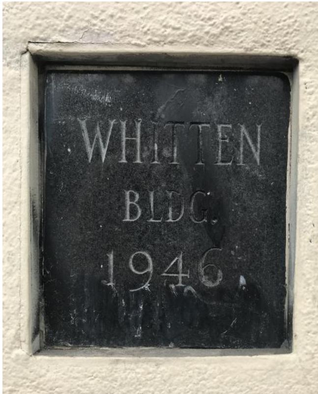
Detail of "corner stone" at lower right side of primary facade.
