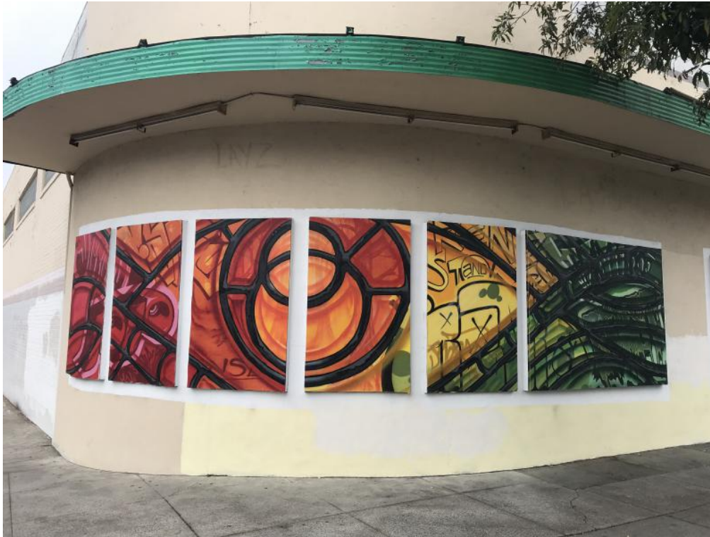
Detail of rounded southeast corner, including punched window openings and awning.
