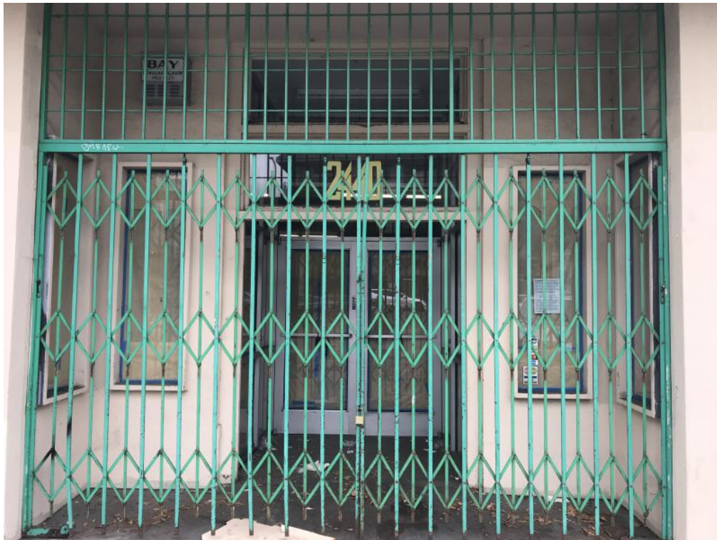
Detail of primary entrance, east facade.
