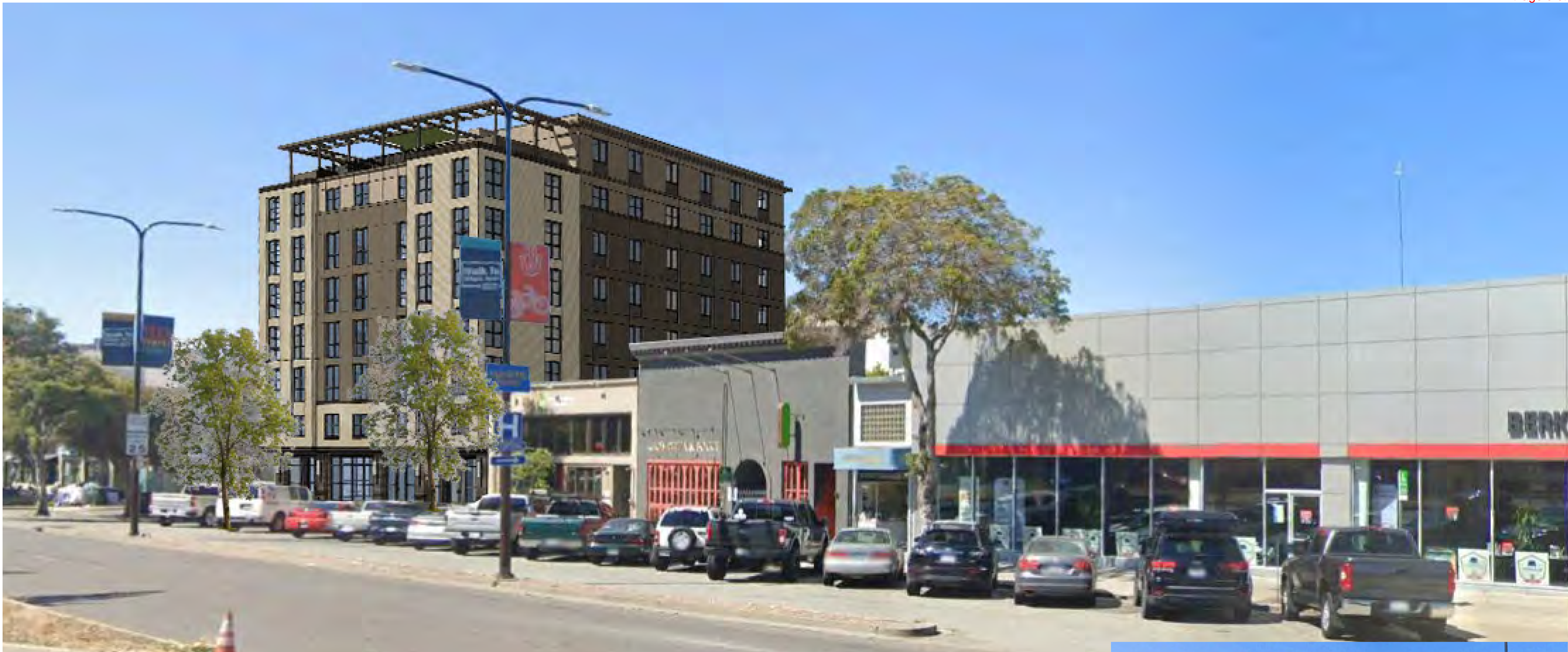
View Looking South West from Shattuck Avenue
