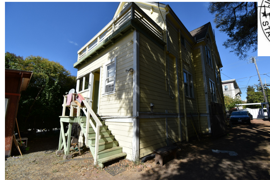
D - EXISTING REAR STAIRWAY
