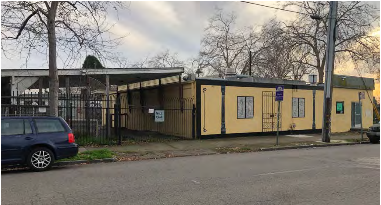
Fig.5 – 2403 San Pablo Ave. - Rear (center) and north side (right), looking south
