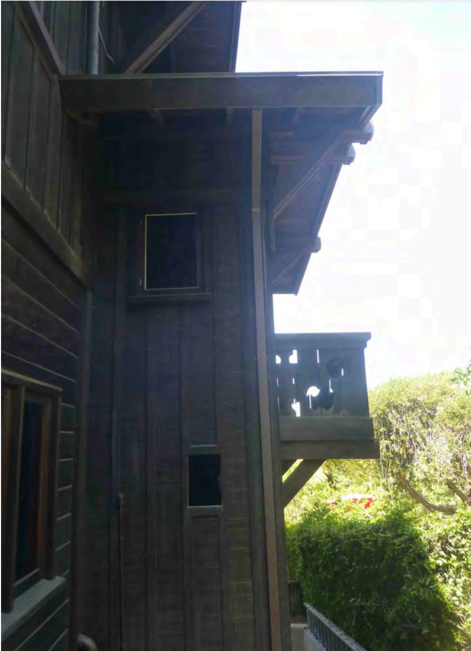
(At left, looking west, along the north wall of the original house, showing the one and a half story board and batten bay that contains the stairwell. The “Juliet” balcony is on the right, and there is a small hipped roof over the projecting bay. Photo S. Finacom, 2021.)
