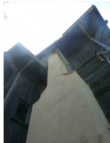
(Above, upper exterior wall and roof detail of north elevation of main house. Note the wide eaves, brackets, board and batten on upper floor, horizontal board siding on main floor, and wooden “posts” expressed on the exterior. This is looking southwest, towards the upper portion of the second floor, with the stairwell bay at right. Photo S. Finacom, 2021)
