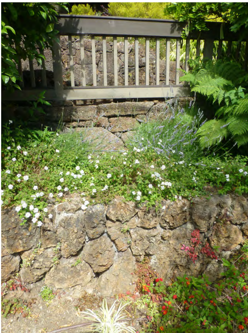
The picture above shows an early, most likely Berkeley Rhyolite, stone wall at the sidewalk edge, with a planter bed above and a newer stone wall, topped by a newer fence, above that. Beyond the fence is yet another section of stone wall. Photo S. Finacom, 2021.)
