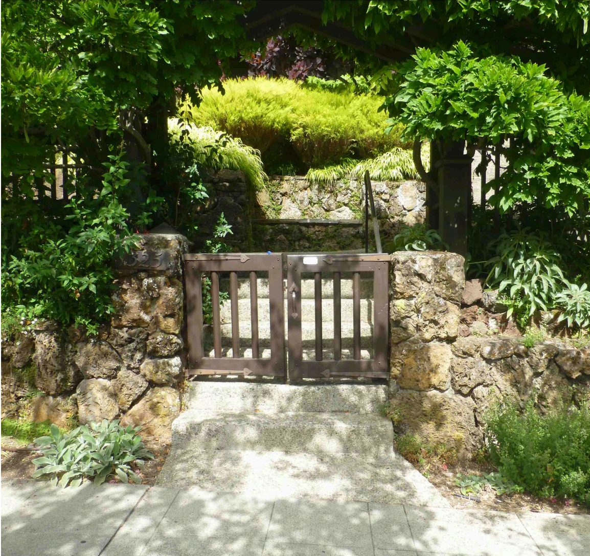
(At right. Entry gate from the street. Stone columns and rhyolite stone walls are from the Period of Significance. Gate and arbor above it are more recent additions, as are concrete stairs. Photo S. Finacom, 2021)
