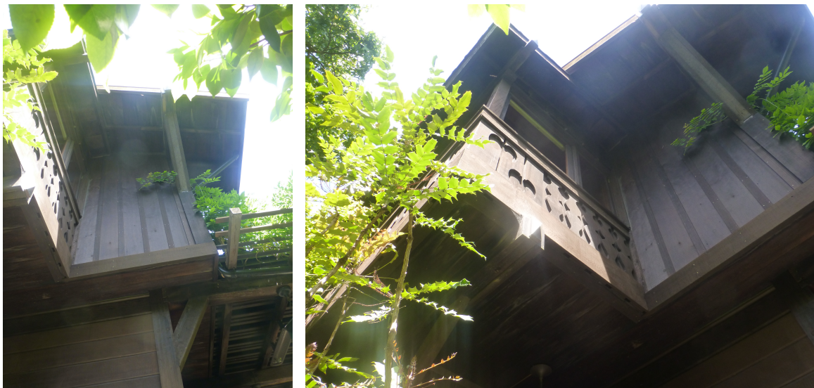
(Above, left and right. Two views of the east end of the sunroom porch and south wall of the house, above the main entry porch / door. Photos S. Finacom, 2021)
