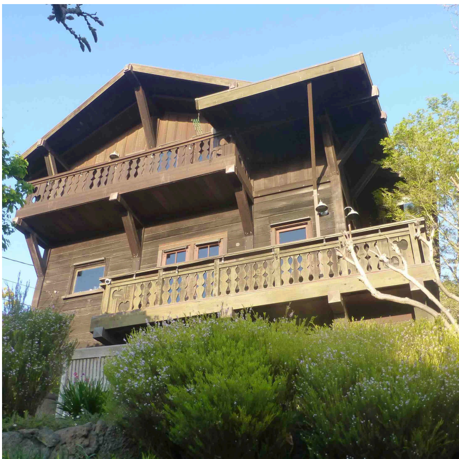
(At left, west elevation showing upper two floors and roof form. Photo S. Finacom. 2021)
