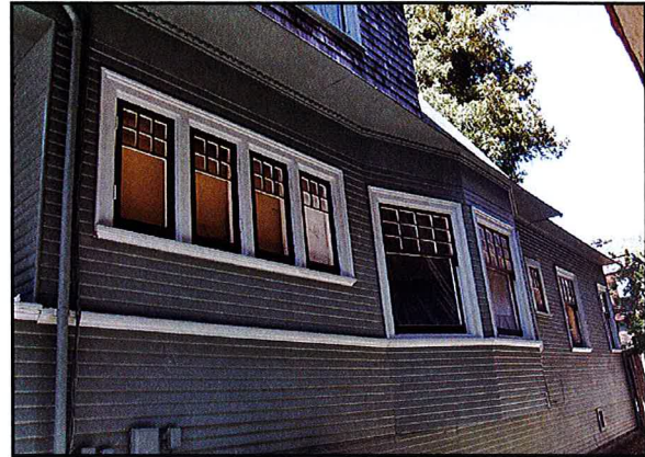
Fig. 10. South façade, looking east. Daniella Thompson, 2021
