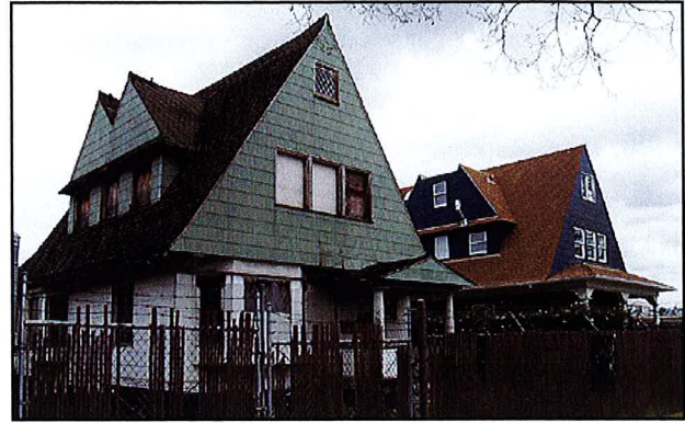
Fig. 26. Snyder House, 2820 San Pablo Ave., designed by A. W. Smith in 1901. Daniella Thompson, 2005.
