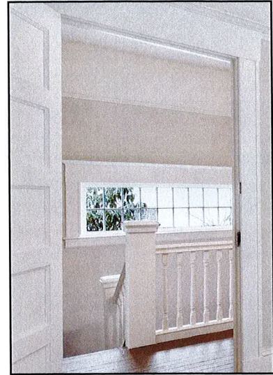
Fig. 12. The stair landing window in the north dormer (before interior demolition) The Grubb Company listing photo, 2021
