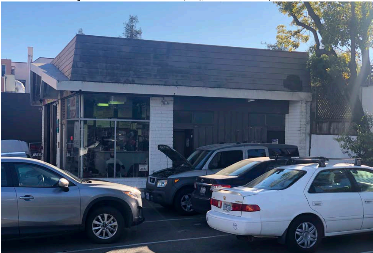
Fig.6 – 1752 Shattuck Ave. – North side, from Francisco St. (MH 2022)
