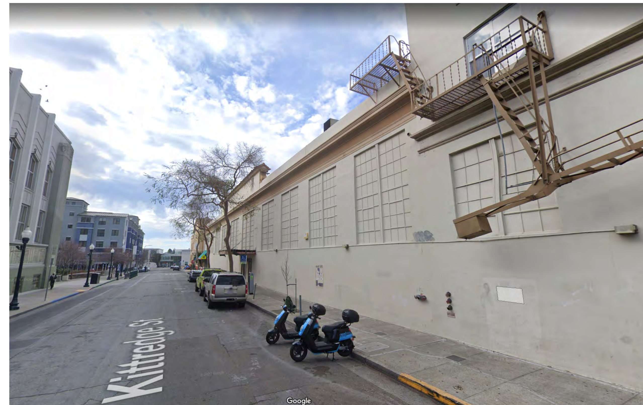
4 SITE PHOTO - KITTREDGE ST - LOOKING WEST A0-001 12" = 1'-0"
