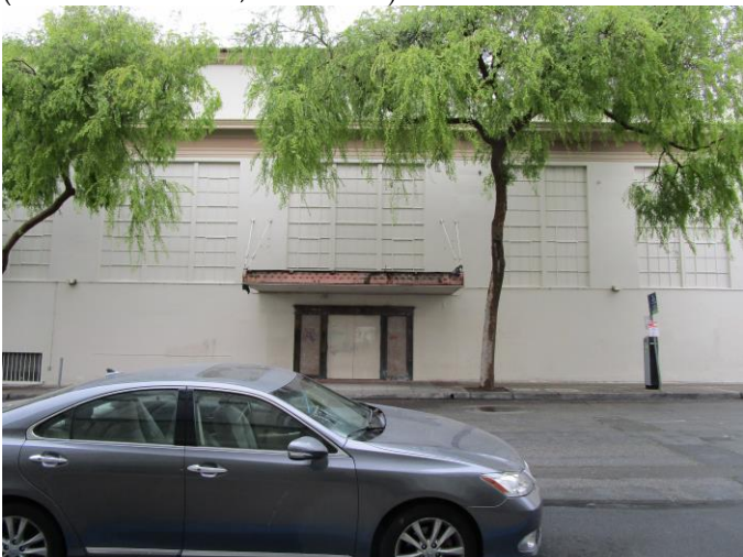
South elevation across Kittridge, view north. (Rincon Consultants, March 2022).
