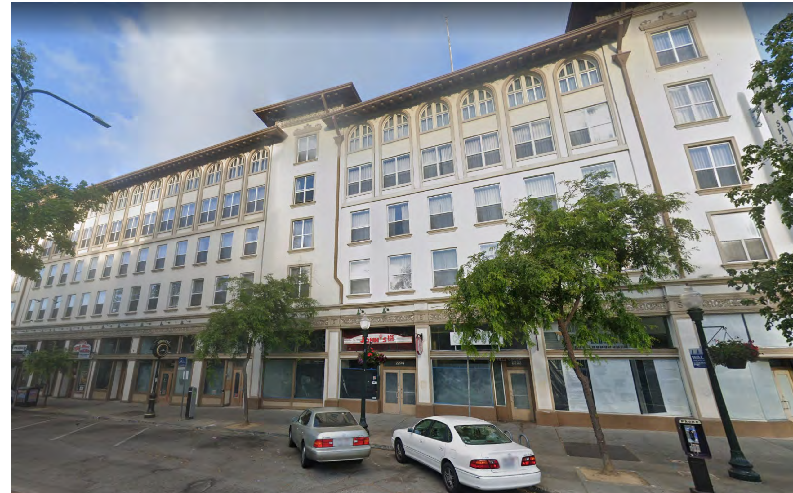
2 SITE PHOTO - SHATTUCK AVE - EXISTING HOTEL AD-003 12" = 1'-0"
