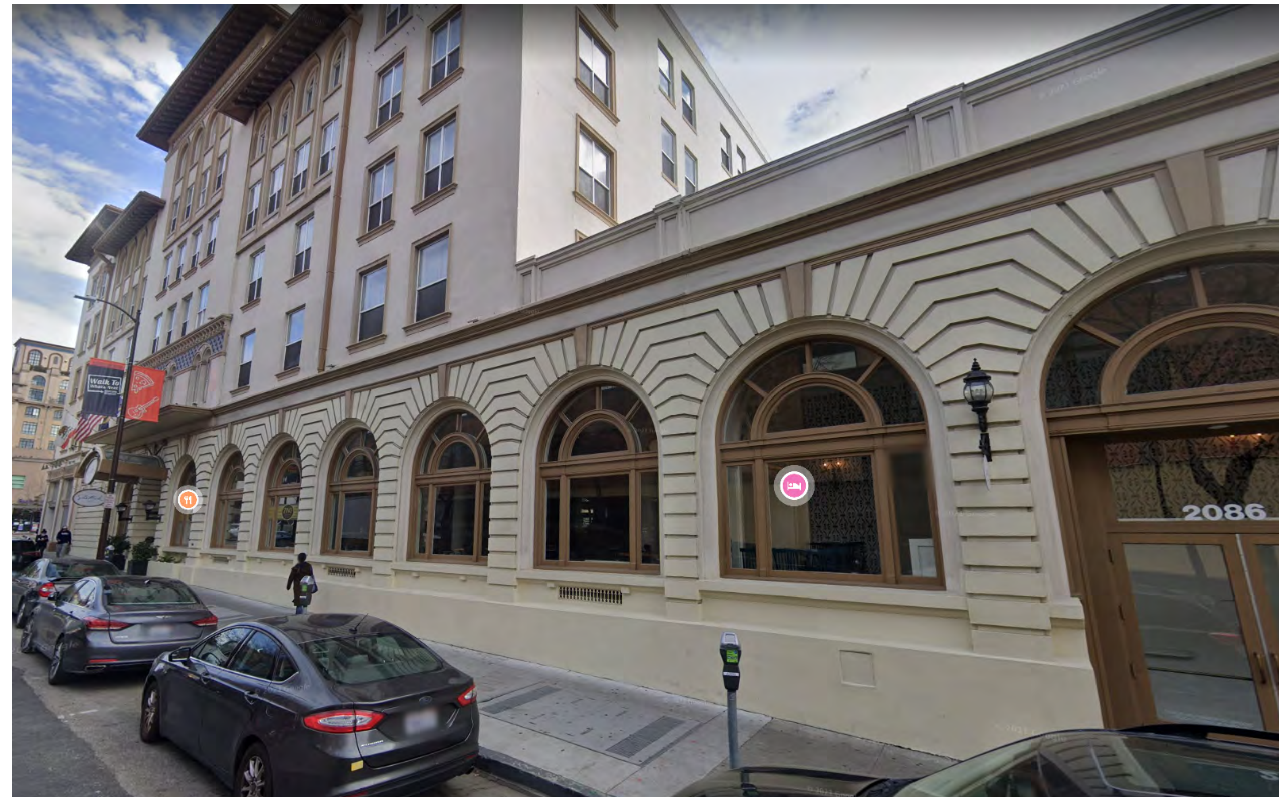
1 SITE PHOTO - ALLSTON WAY - EXISTING HOTEL AD-003 12" = 1'-0"
