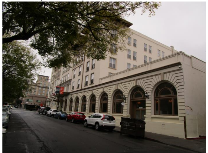
North elevation, view southeast. (Rincon Consultants, March 2022).
