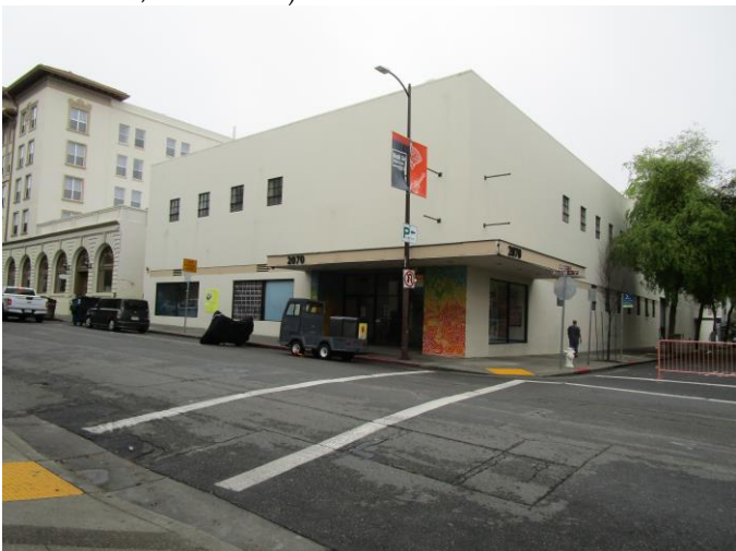
North elevation with Hink's Building (non-contributing) in foreground, view southeast. (Rincon Consultants, March 2022)
