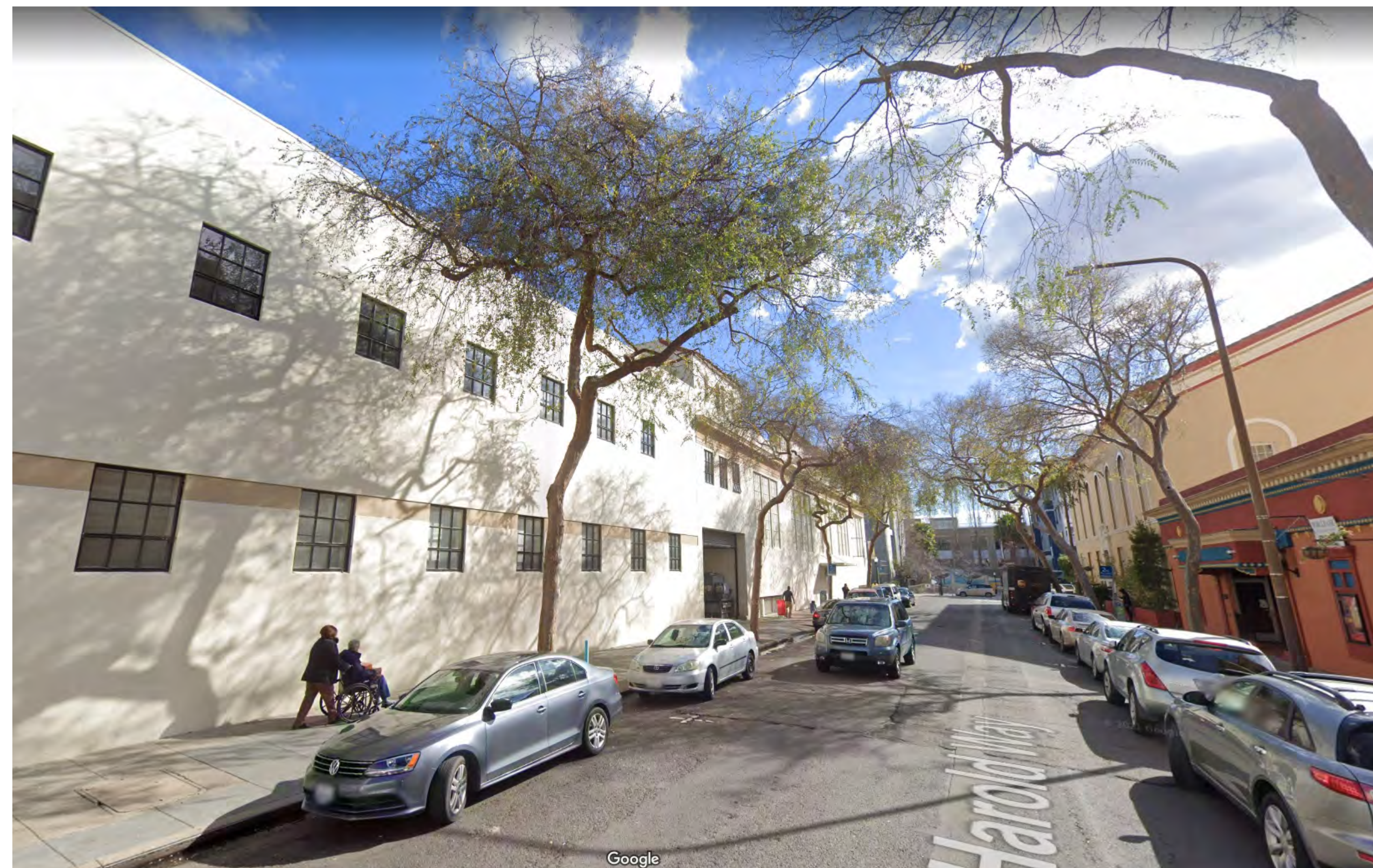
3 SITE PHOTO - HAROLD WAY - LOOKING SOUTH A0-001 12" = 1'-0"
