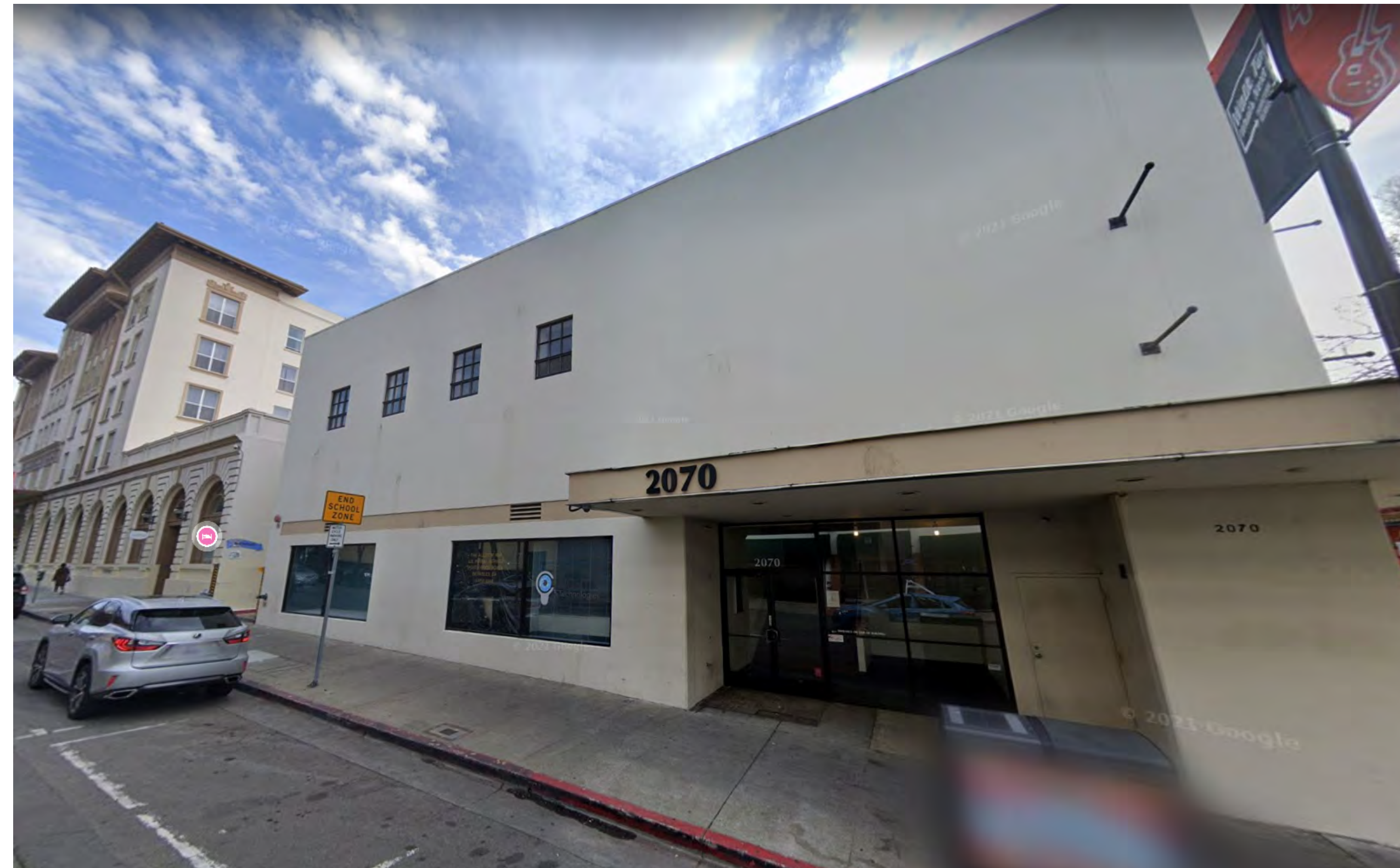
1 SITE PHOTO - ALLSTON WAY FACADE A0-002 12" = 1'-0"
