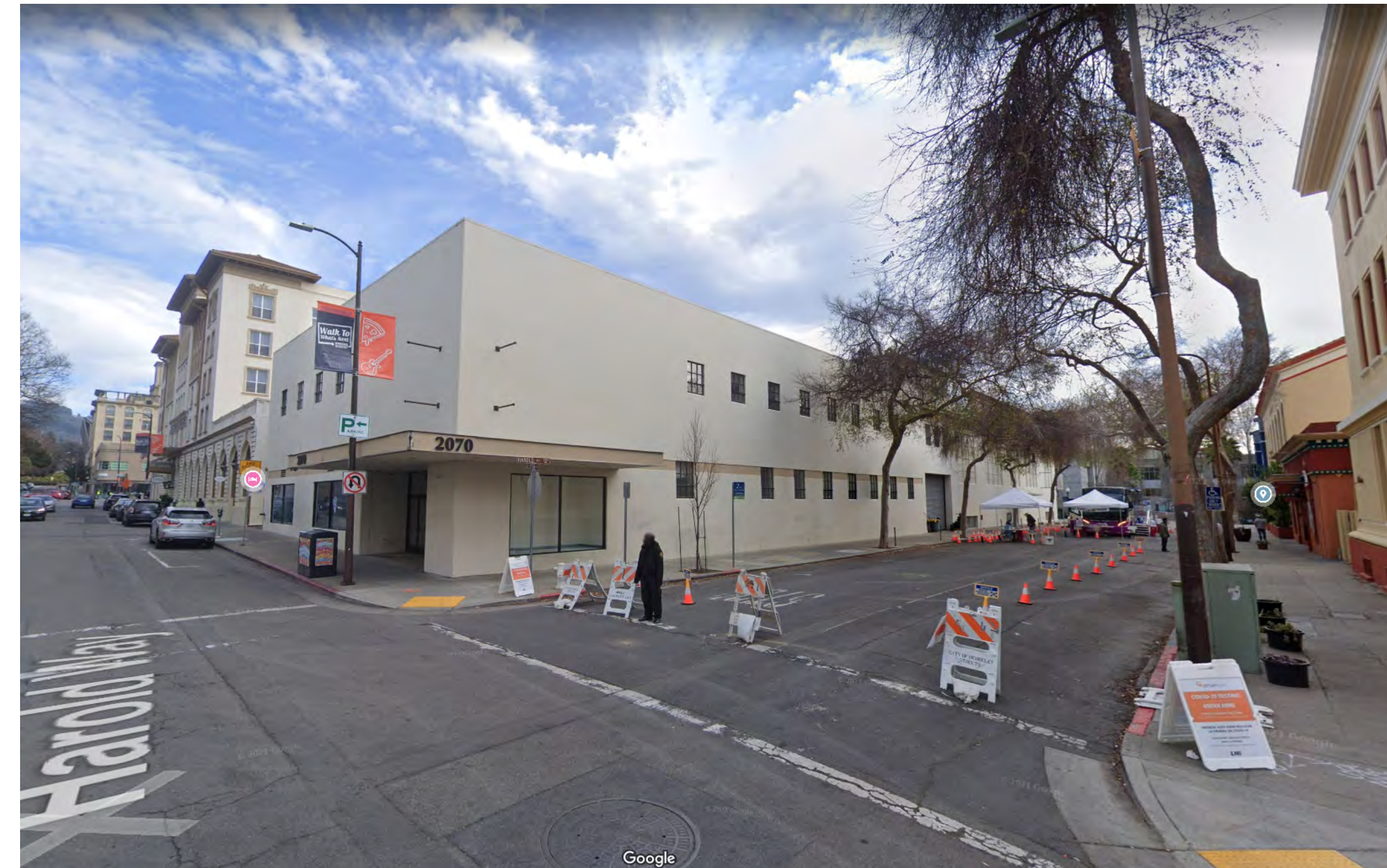
2 SITE PHOTO - ALLSTON WAY AND HAROLD WAY - LOOKING EAST A0-001 12" = 1'-0"
