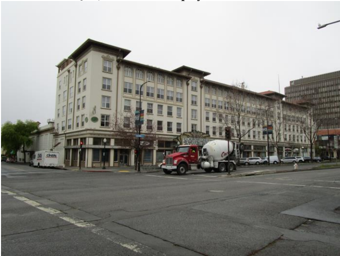
Shattuck Hotel, south and east elevations, view northwest. (Rincon Consultants, March 2022)
