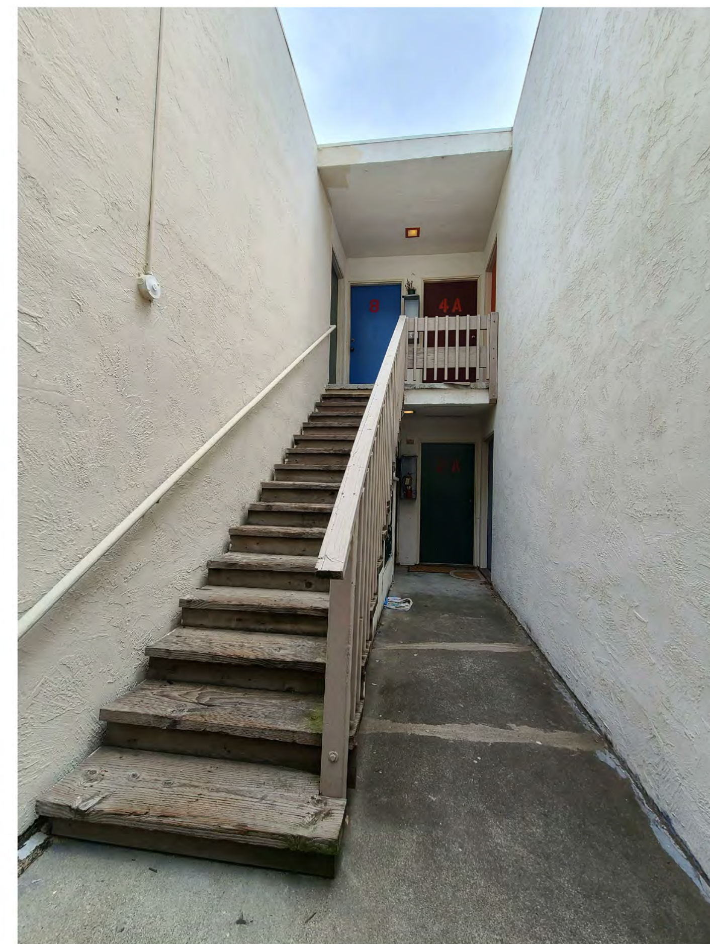
6 EXISTING APARTMENT STAIR, WEST SIDE G003 1/2" = 1'-0"
