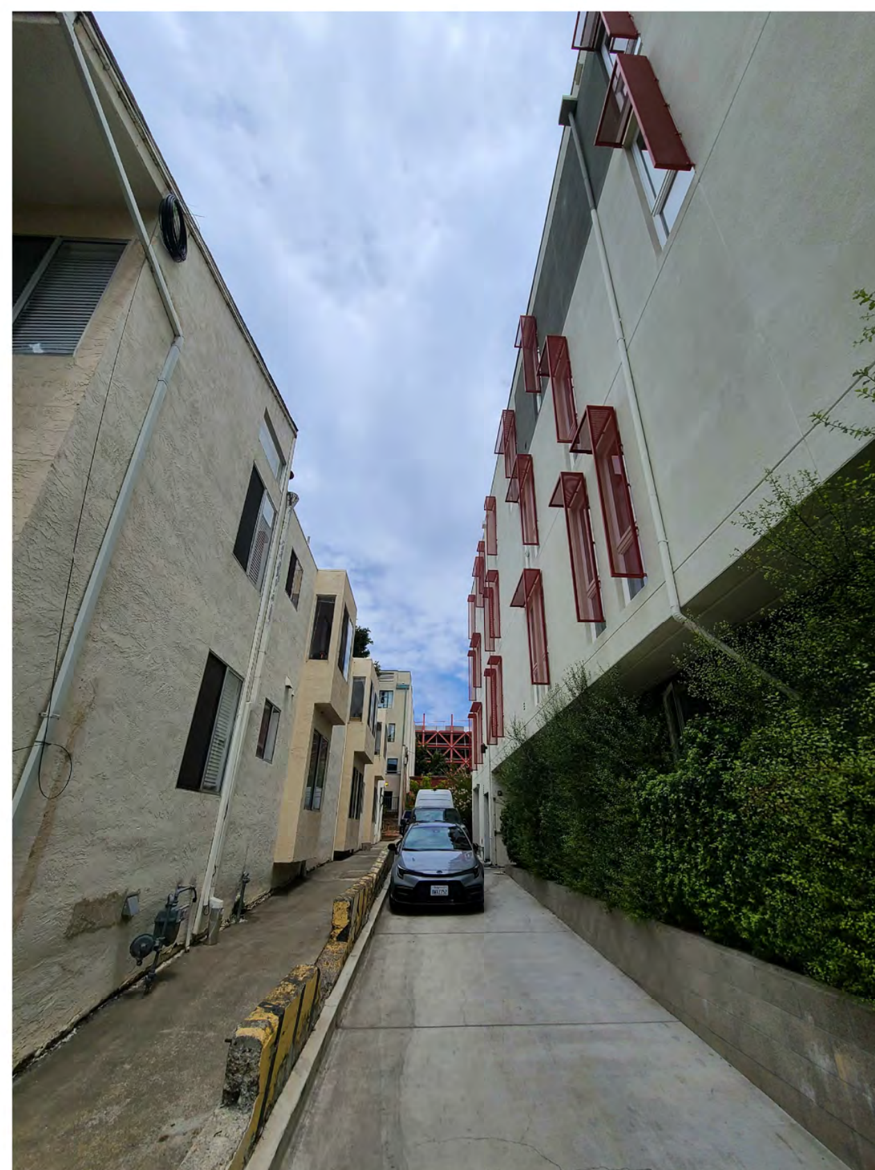
3 EXISTING SIDE YARD, EAST SIDE LOOKING NORTH G003 1/2" = 1'-0"
