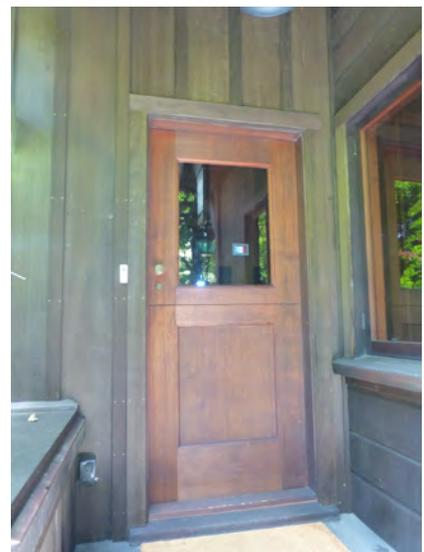
the kitchen originally projected a short distance—a little over eight feet—forming a small extension, less than ten feet wide, clad in vertical boards and battens, on the northeast corner of the house. The kitchen extension contained a small window on the south (left) and a back door on the right (north). The design of the back door is not indicated on the original plans, but it was covered on the exterior by a screen door divided into upper and lower panels.
