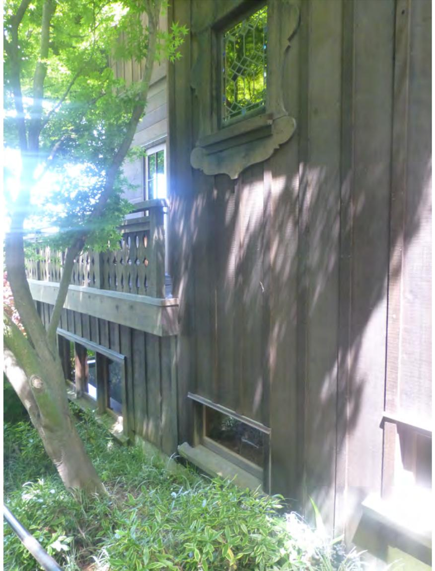
The original drawings show two windows in this location, slightly divided by a section of wall. Further east on the wall there is a horizontal, single-lite, window with obscure glass. This appears to be an addition, since the original working drawings show only a small opening in this area, perhaps a ventilation grate or hatch.
