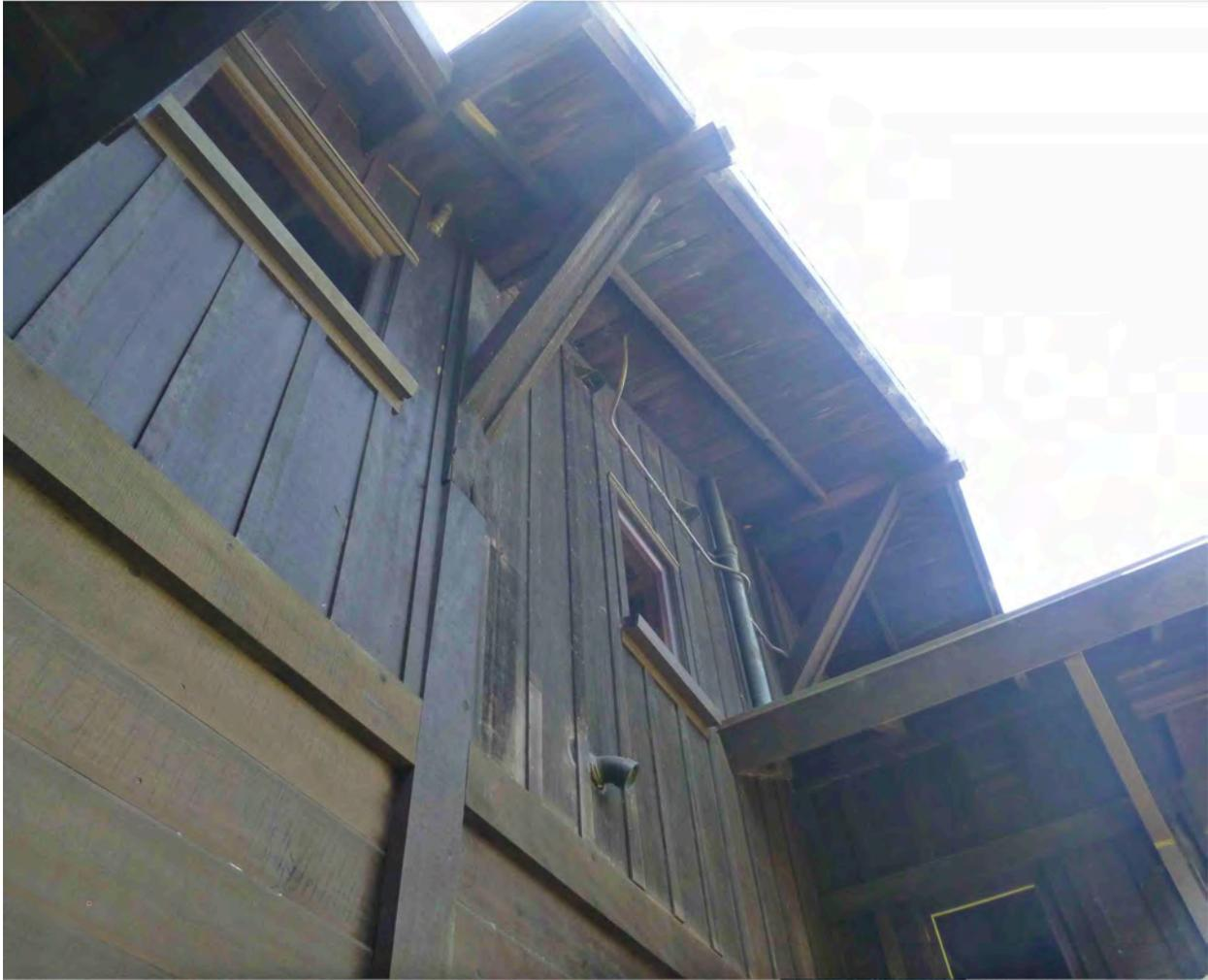
*(Above, upper exterior wall and roof detail of north elevation of main house. Note the wide eaves, brackets, board and batten on upper floor, horizontal board siding on main floor, and wooden “posts” expressed on the exterior. This is looking southwest, towards the upper portion of the second floor, with the stairwell bay at right. Photo S. Finacom, 2021)*
