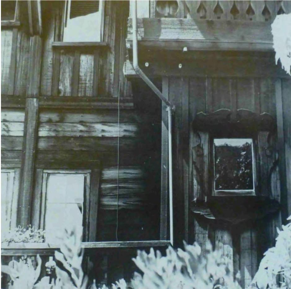
*(At left. 1970s photograph of south facade, showing deteriorated horizontal board siding at first floor level, original French doors from living room to balcony at left, and original scroll-sawn wooden surround for vestibule window, at right. Source: Freudenheim.)*
