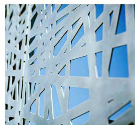
PERFORATED METAL PANEL AT BALCONY RAILING
