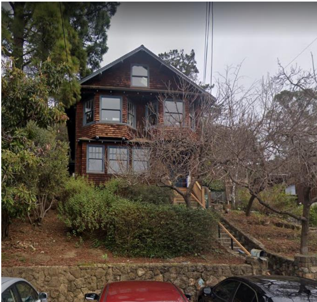
Figure 2: Subject Building, Existing Site Conditions (Google streetview, 2021)
