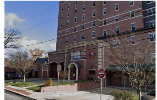
Lincoln Towers in Wilmington, DE
