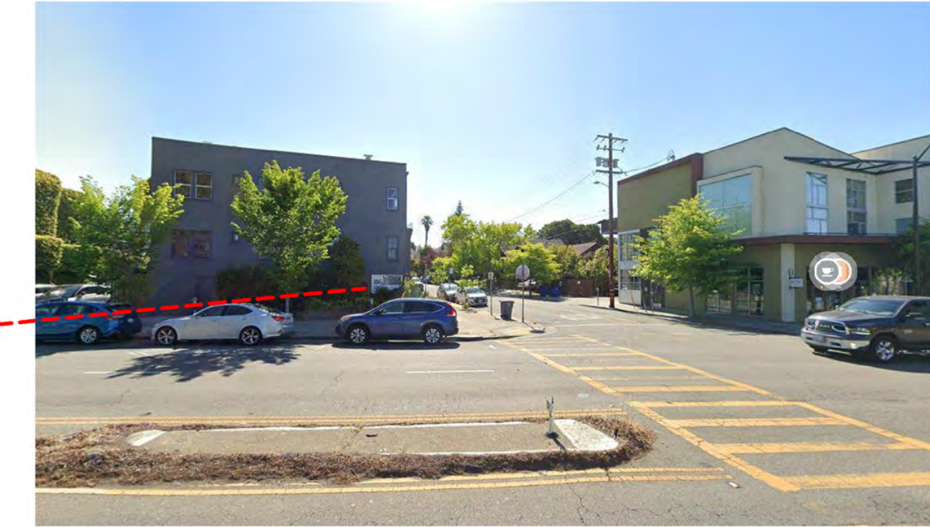
3045 & 3085 TELEGRAPH AVE. - RESIDENTIAL & MIXED-USE BUILDINGS
