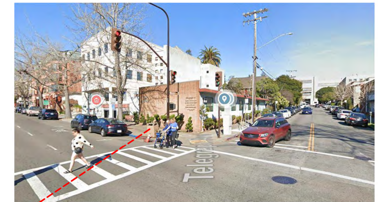
3021 & 3017 TELEGRAPH AVE. - COMMERCIAL BUILDINGS
