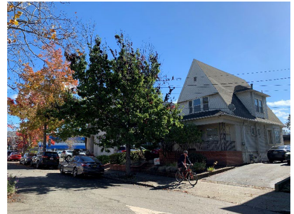
The existing four units will be replaced within the project
