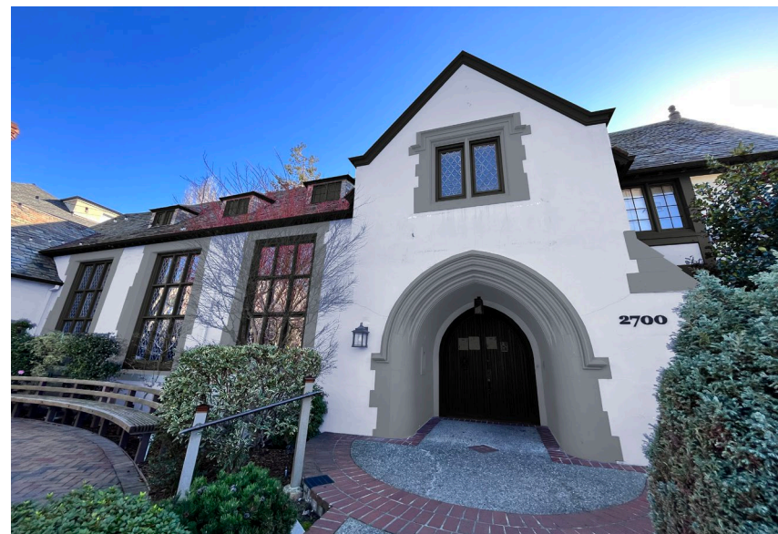
EXTERIOR STREET VIEW HERITAGE HOUSE SCHEME B
