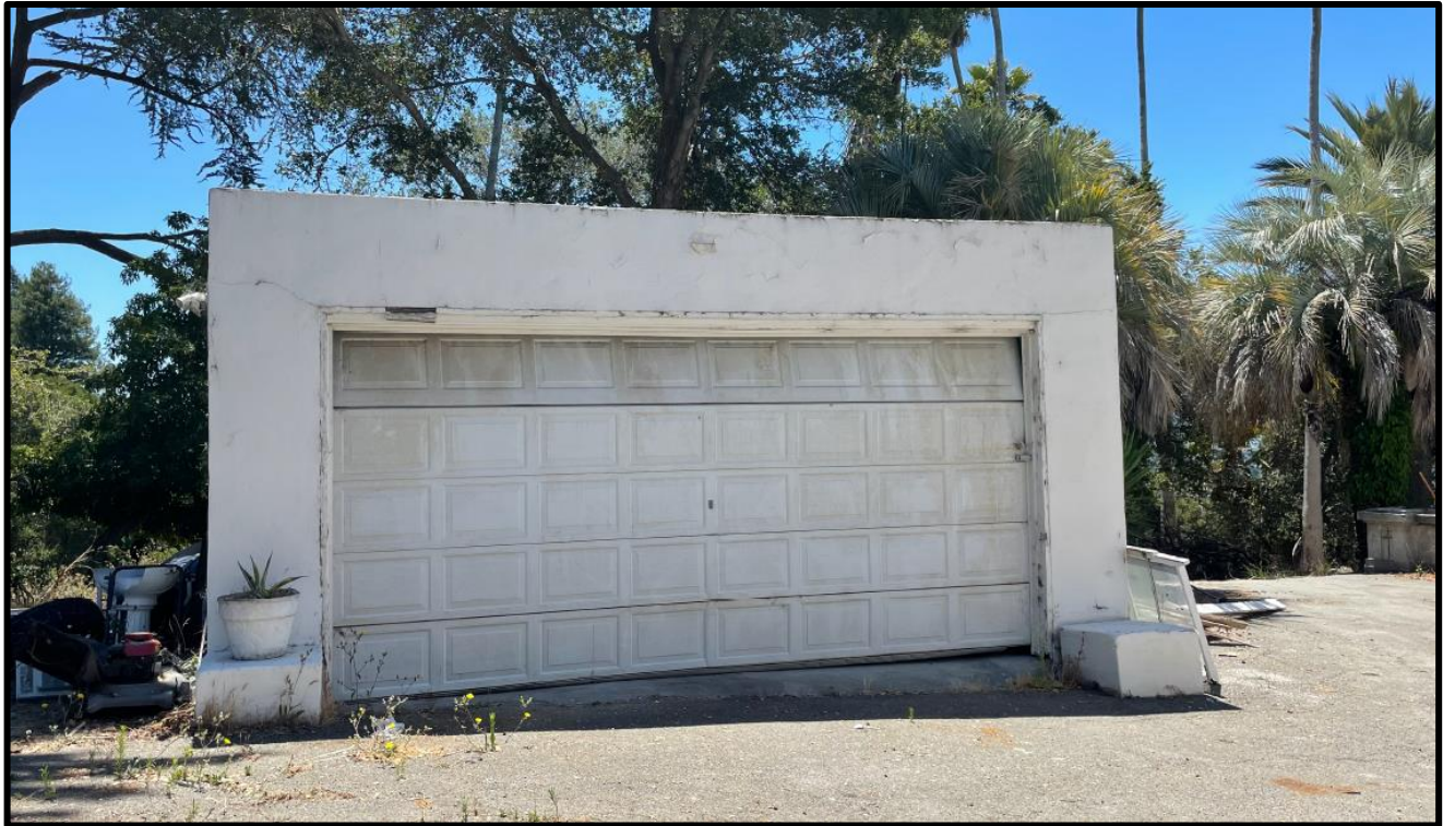
Figure 4: Subject property, north elevation of garage to be demolished (2022).
