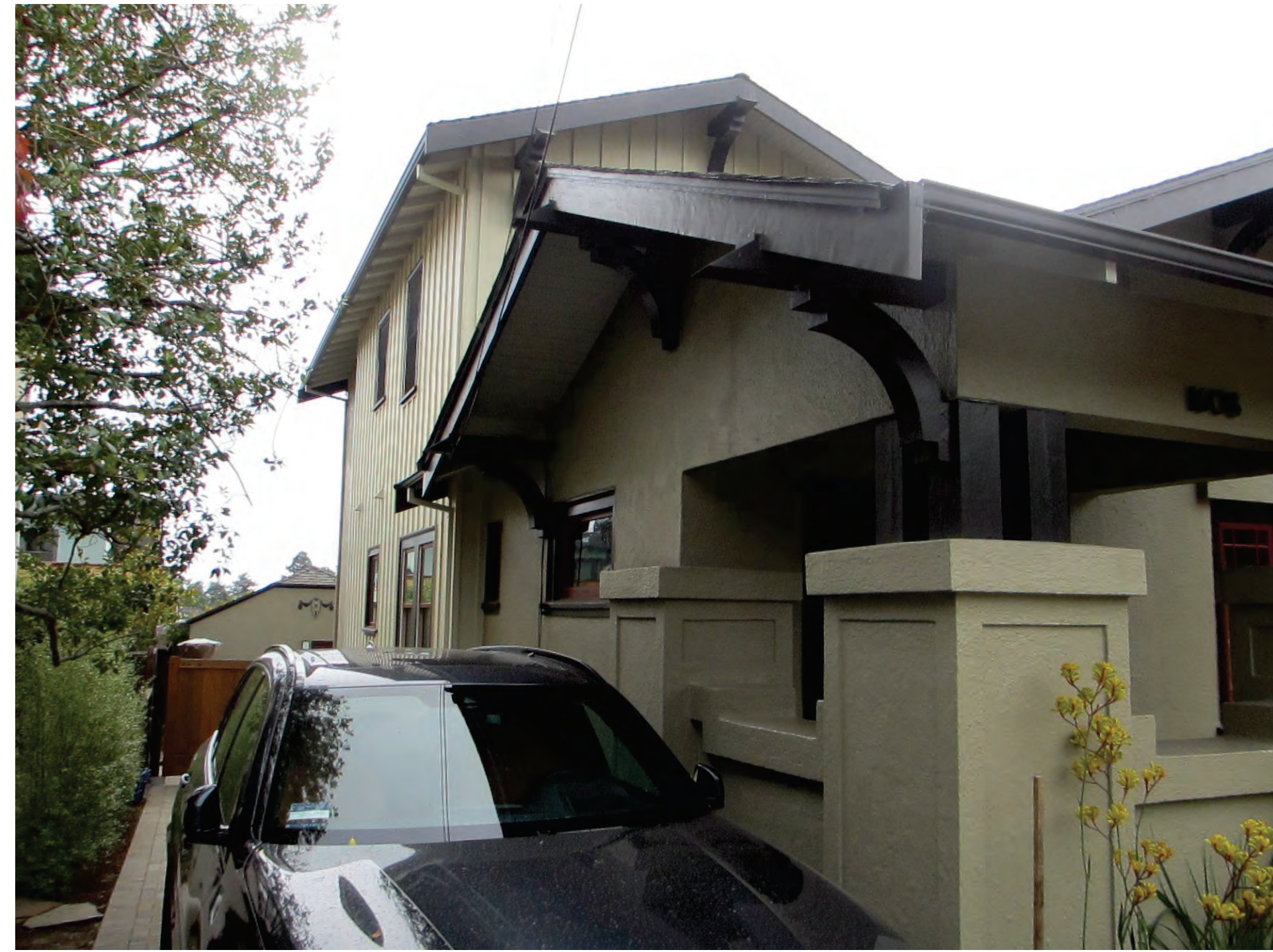
7 EXISTING HOUSE - FRONT/SIDE (NORTHEAST)
