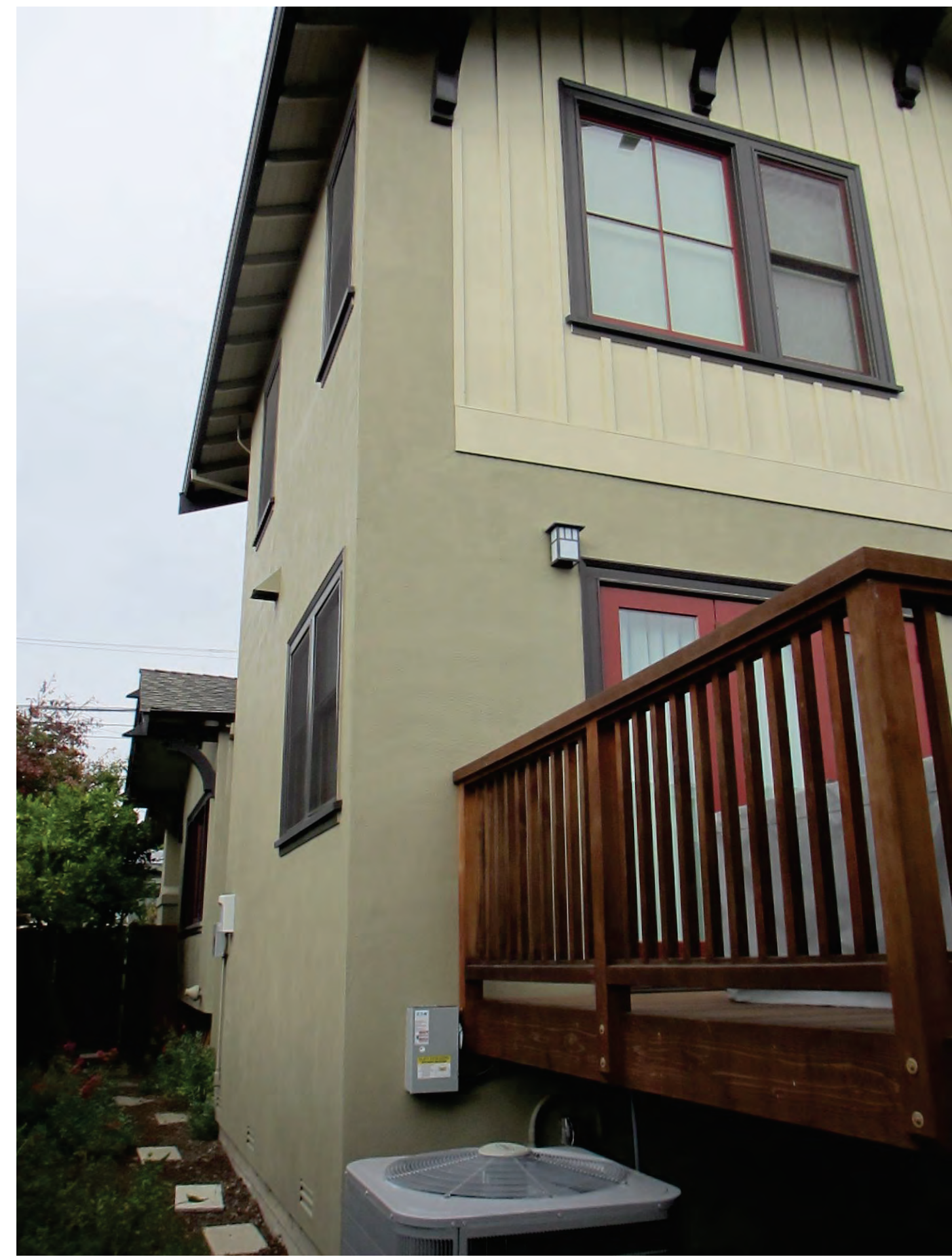
3 EXISTING HOUSE - REAR (SOUTHWEST) ELEVATION
