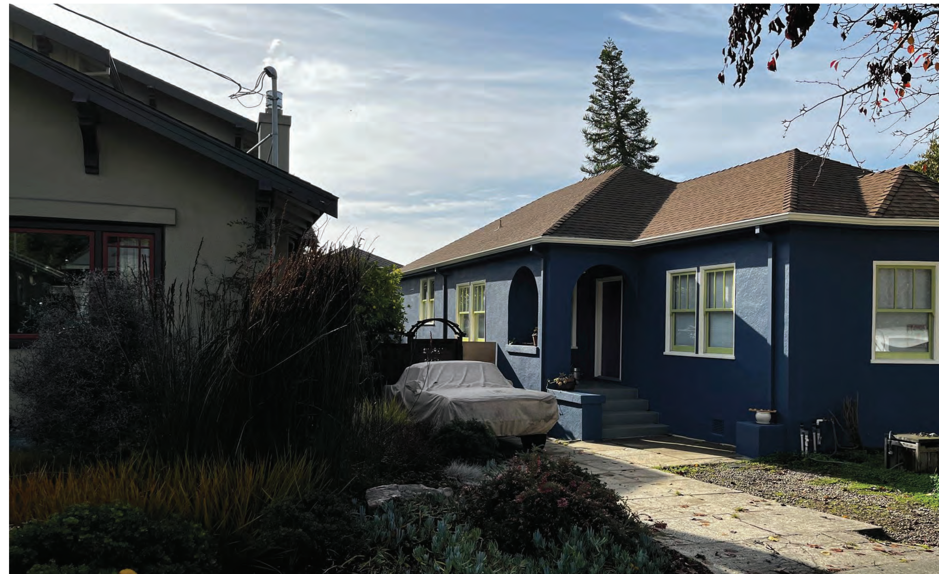
3 WINTER (12/28) AT NOON - 1604 BEVERLY PL. (PHOTOGRAPH) EXISTING BUILDING
