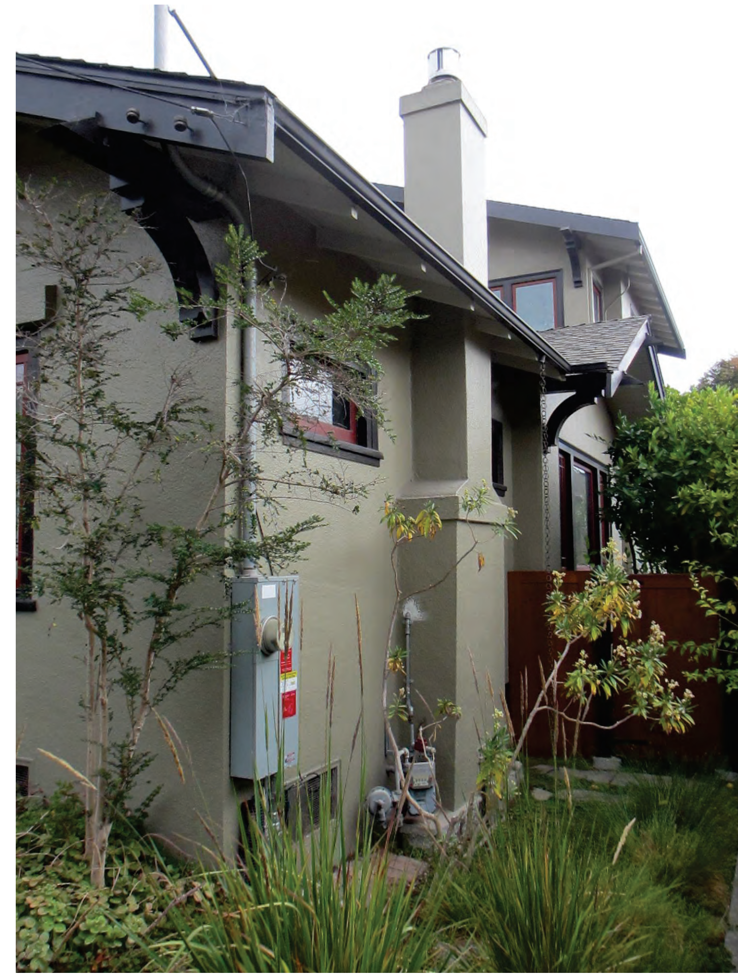
5 EXISTING HOUSE - FRONT/SIDE (NORTHWEST)
