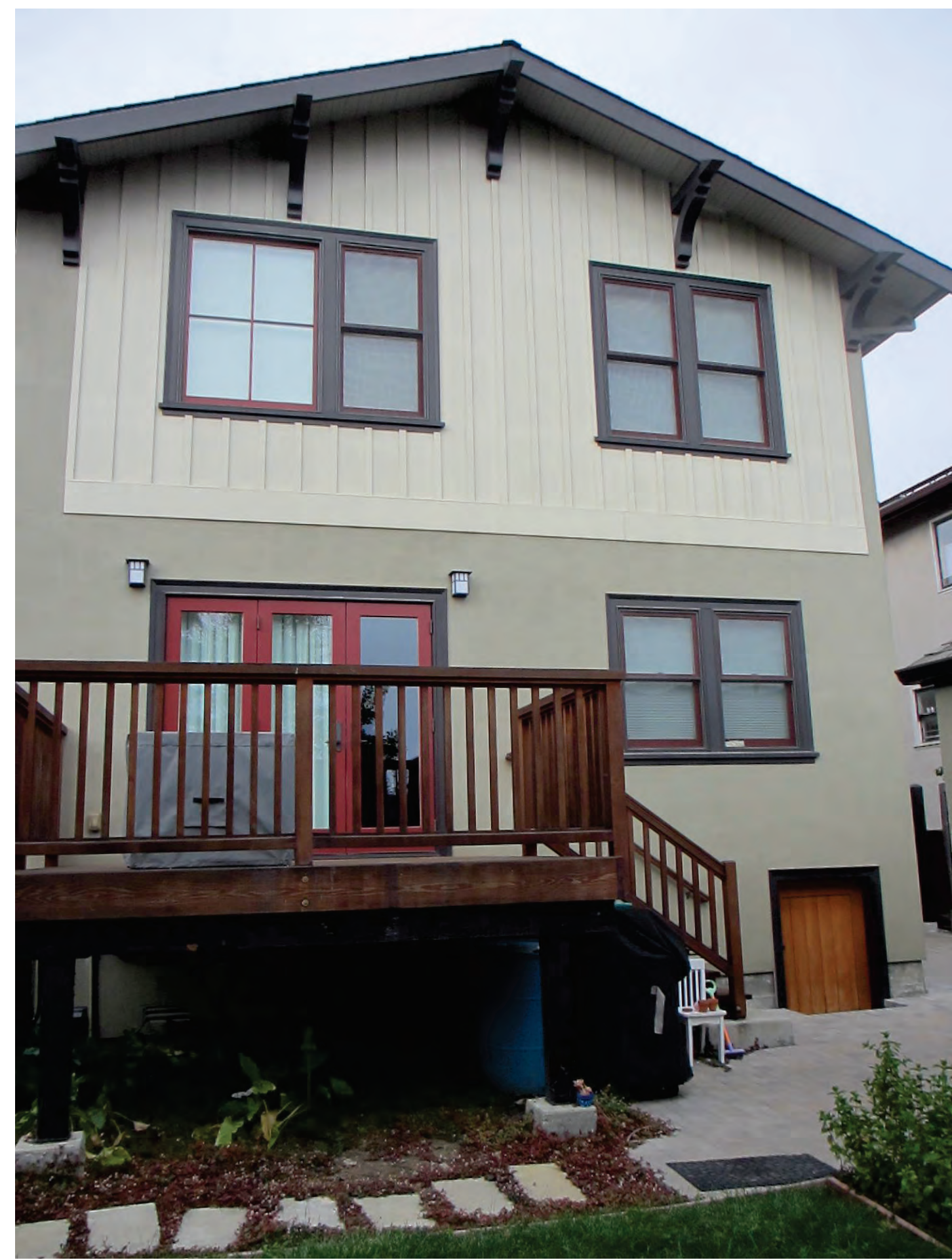
2 EXISTING HOUSE - REAR (SOUTH) ELEVATION
