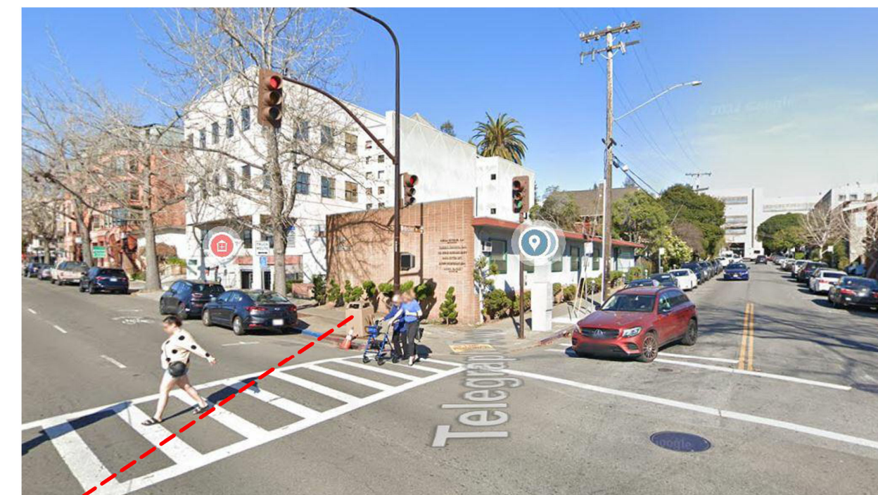
3021 & 3017 TELEGRAPH AVE. - COMMERCIAL BUILDINGS
