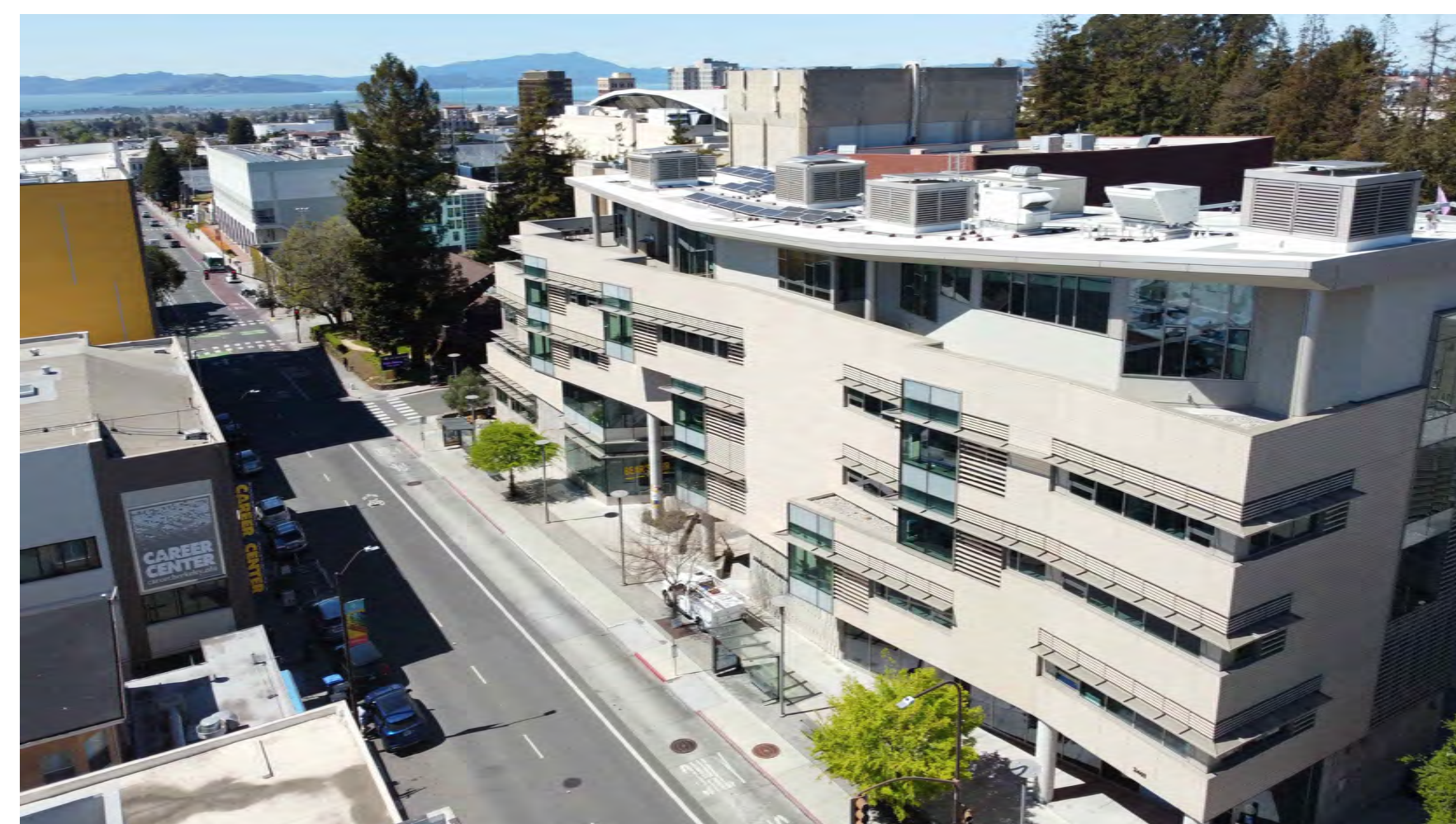
5 VIEW OF EXISTING CONTEXT FACING NORTHWEST FROM PROJECT SITE
