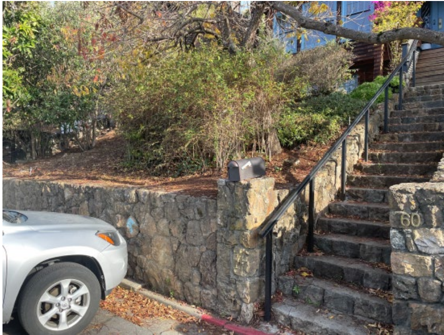
Figure 5: Subject property, stone retaining wall at front property line in 2022 (Kanarek)
