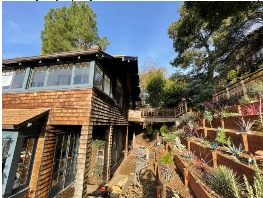
Figure 4: Subject property, south and west elevations in 2022 (Kanarek)
