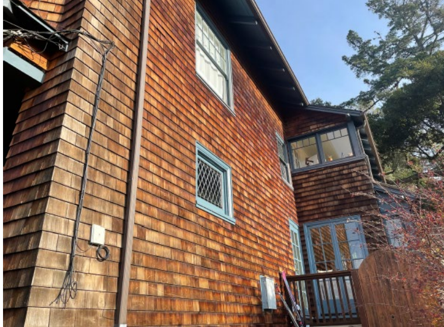
Figure 3: Subject property, north elevation in 2022 (Kanarek)
