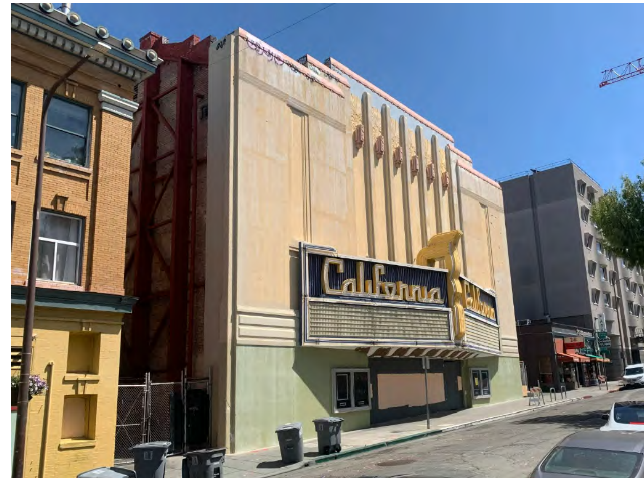
2 STREET VIEW LOOKING NORTH
