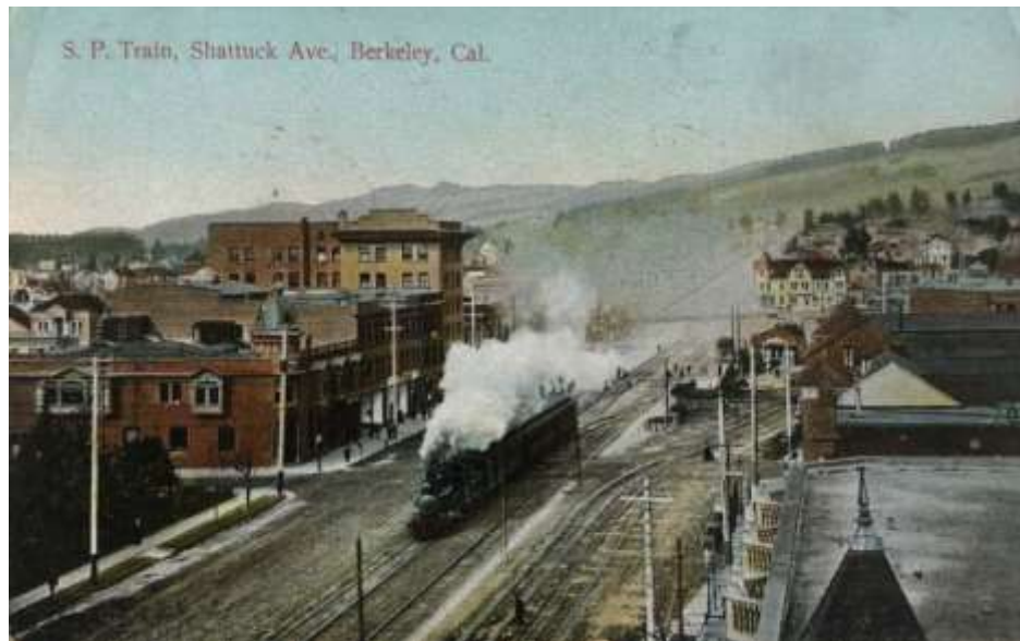
Figure 9. Southern Pacific station on Shattuck Avenue, circa 1909
