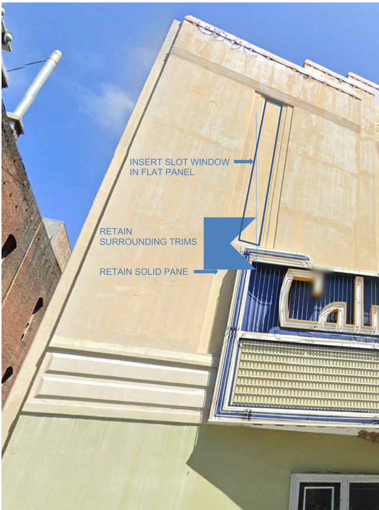
Fig.6 – California Theatre – Recommended window treatment
