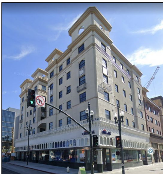
Figure 21: Acheson Commons example (SW Corner)
