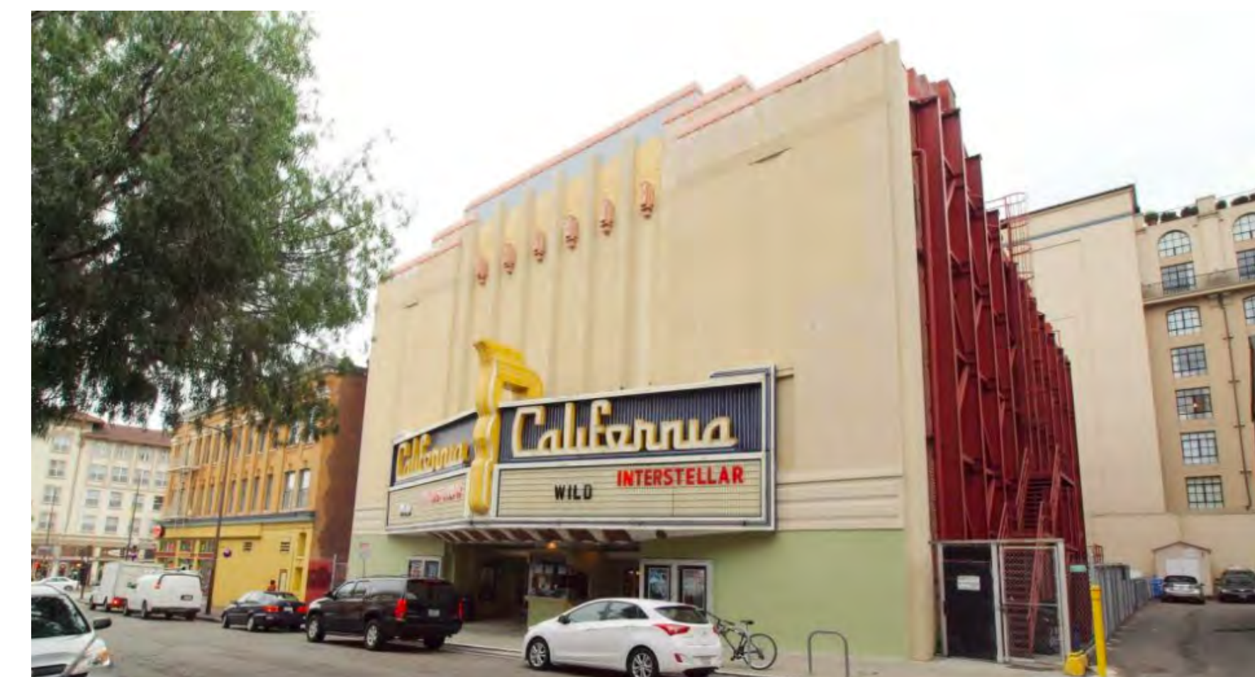
3 STREET VIEW LOOKING WEST
