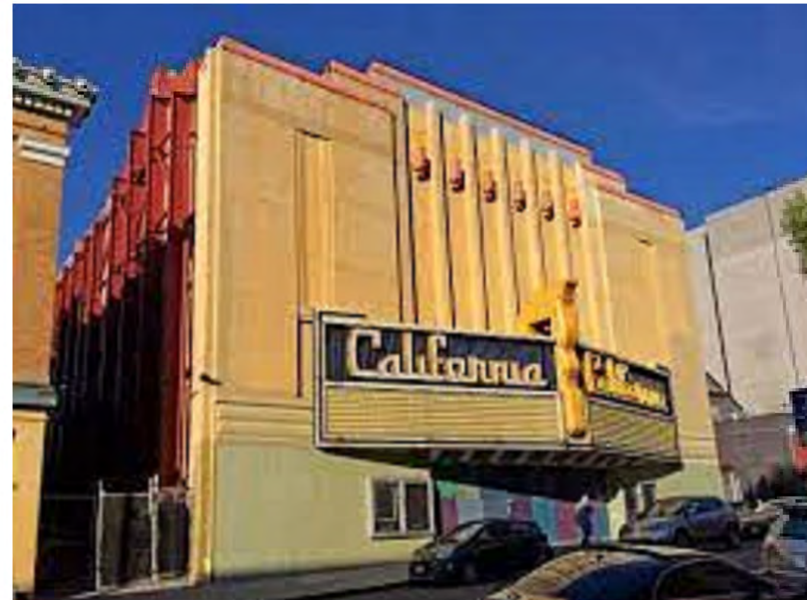
EXISTING THEATER FACADE
