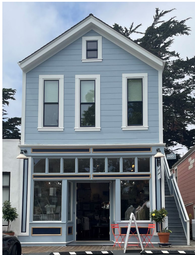
Figure 3: South Façade (Delaware Street), Existing Conditions
