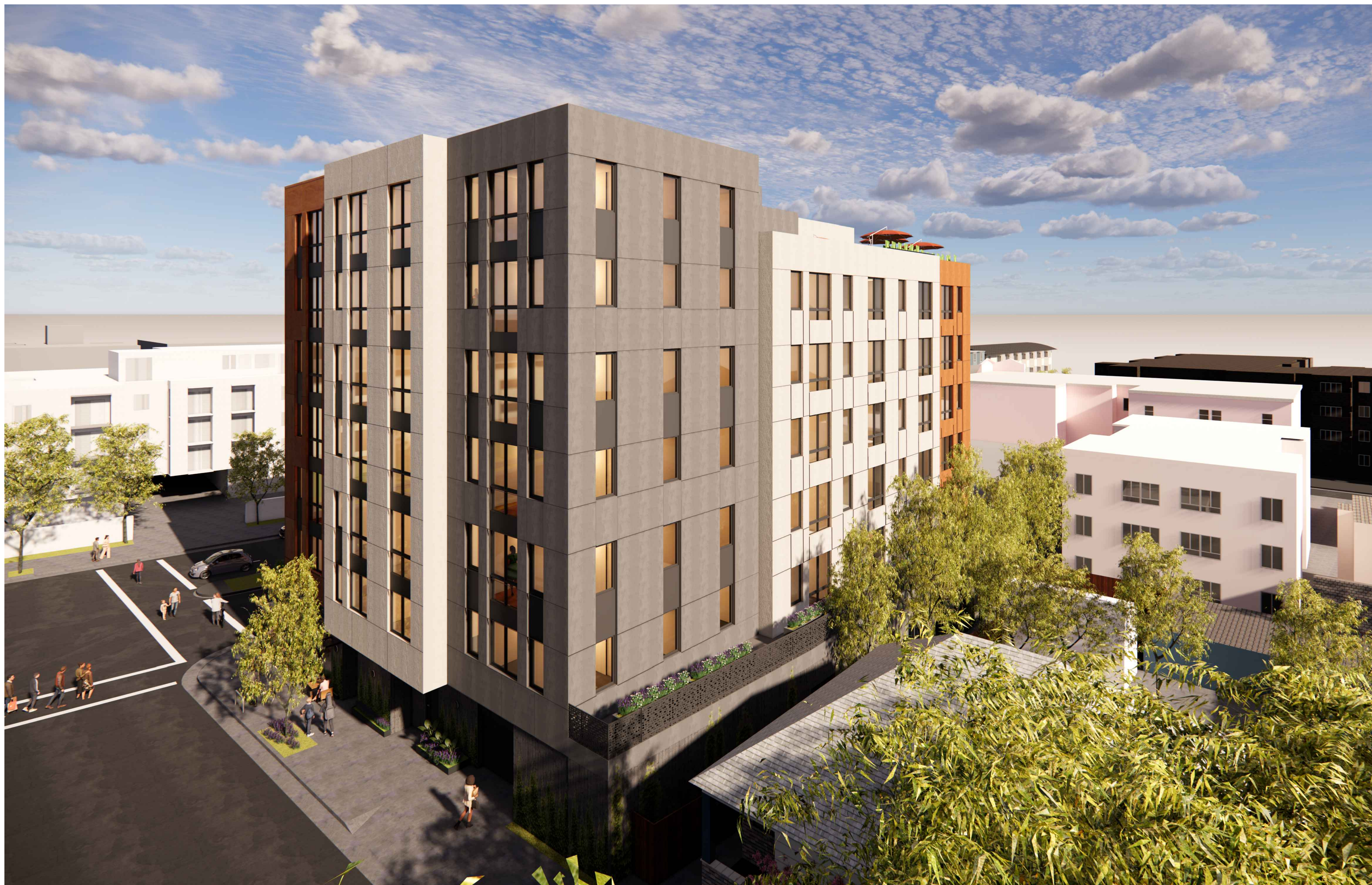
1 - VIEW OF NORTHWEST CORNER
