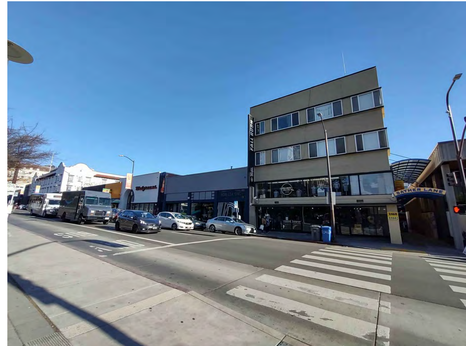
1 VIEW OF EXISTING SITE FACING SOUTHEAST FROM BANCROFT WAY
