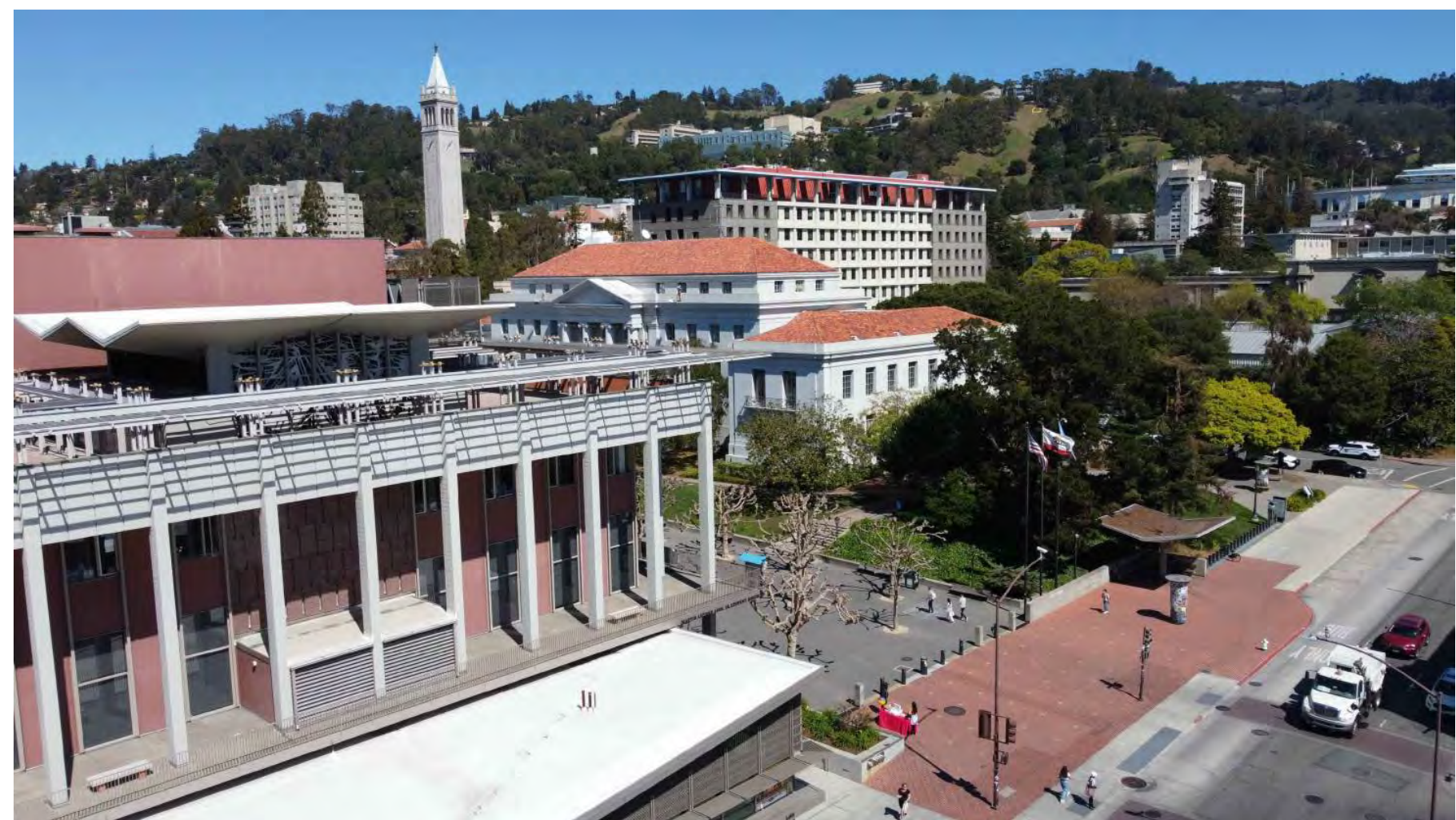
4 VIEW OF EXISTING CONTEXT FACING NORTHEAST FROM PROJECT SITE
