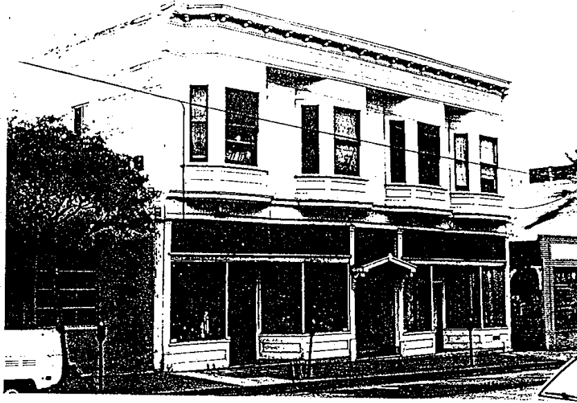
Davis-Byrne Building at 2140 DWIGHT WAY, Dec., 1990
