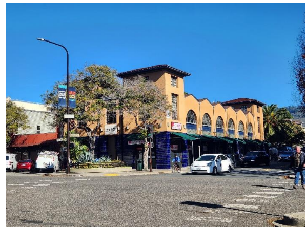
Figure 13: Multi-tenant two-story commercial building at 2395-2399 Shattuck Avenue. Looking northeast.
