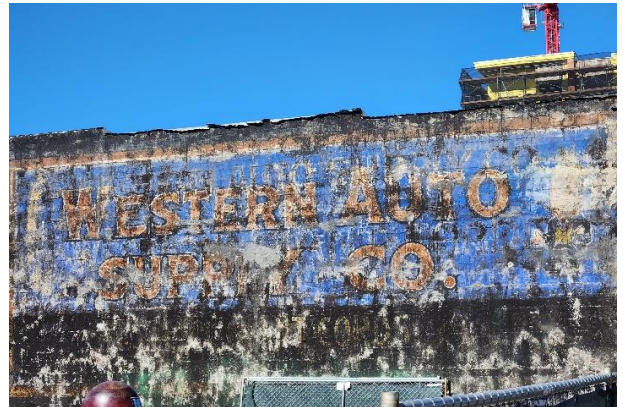
Figure 22: Mural on south façade of 2428 Shattuck Avenue, December 8, 2022.
