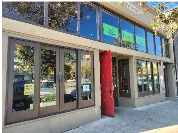
Figure 2: Oblique view of east façade. Looking northwest.
