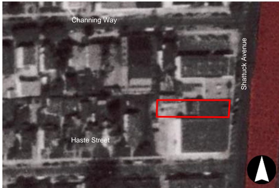
Figure 27. 1947 aerial photograph of Berkeley, showing earliest known footprint of subject building. Subject parcel outlined red. Source: David Rumsey Historical Map Collection.
