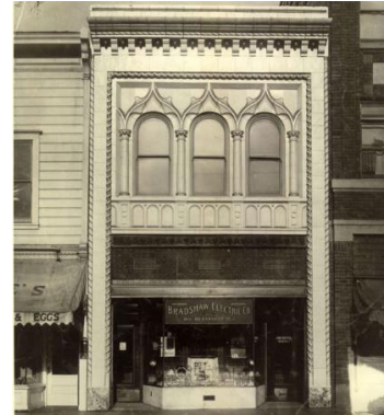
Figure 24: Heywood Building. Designed by James W. Plachek, built in 1917. Berkeley Landmark #181. Source: James W. Plachek Collection, Berkeley Architectural Heritage Society.
