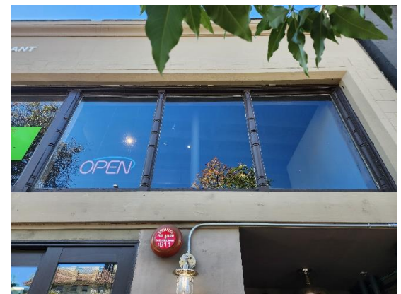
Figure 7: Detail of wood mullions and clerestory at north end of east façade. Looking west.
