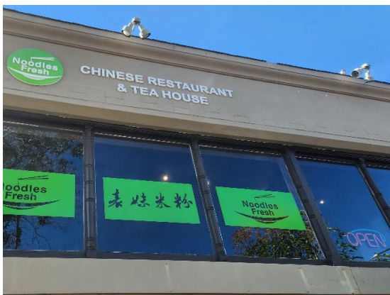
Figure 6: Detail of tenant signage, lighting, and cornice. Looking west.
