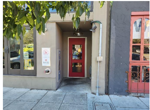
Figure 5: Detail of emergency exit at north end of east façade. Looking west.
