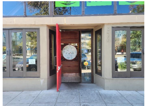
Figure 3: Detail view of primary entrance at east façade. Looking west.
