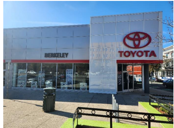
Figure 11: One-story auto dealership north of subject building at 2400 Shattuck Avenue. Looking west.
