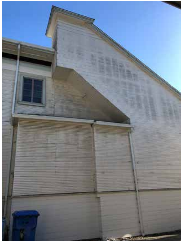
Fig.8 – 2712 Telegraph Ave. – Rear addition at south side
