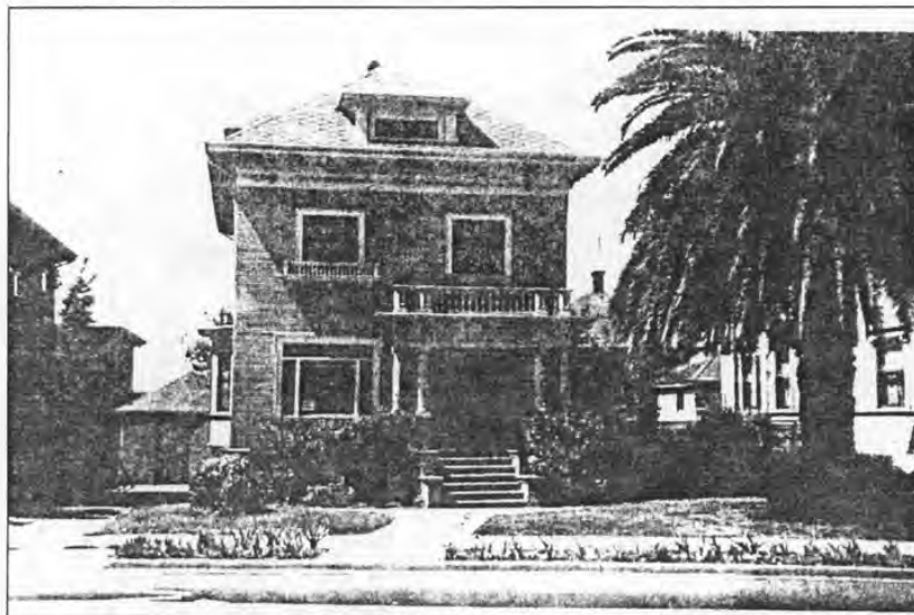
Figure 1. 2712 Telegraph Avenue, 1939 [Ormsby Donogh Collection, Berkeley Architectural Heritage Association]
