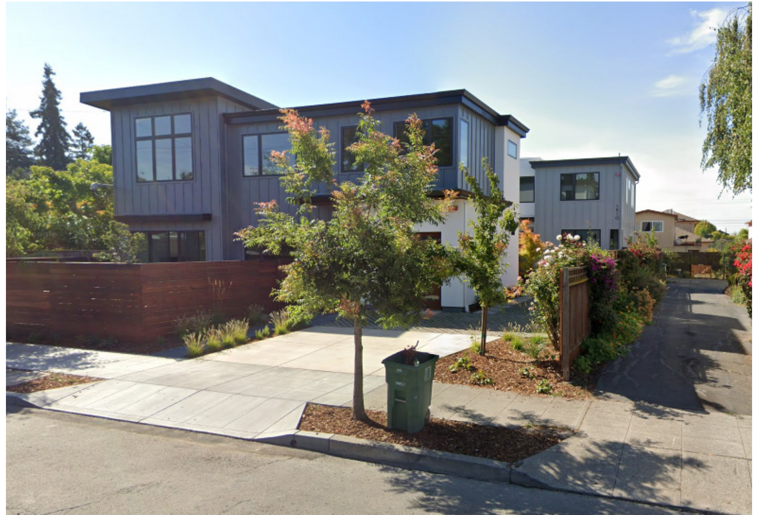
1510, 1512, 1516 CARLETON (LOT DIRECTLY BEHIND PROJECT SITE)
