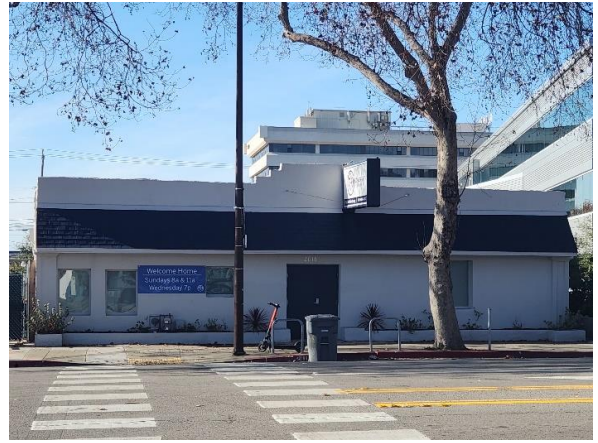
Figure 13: One-story church south of subject building at 2618 San Pablo. Looking west.
