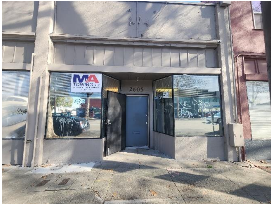
Figure 4: Detail of south storefront on west façade. Looking east.
