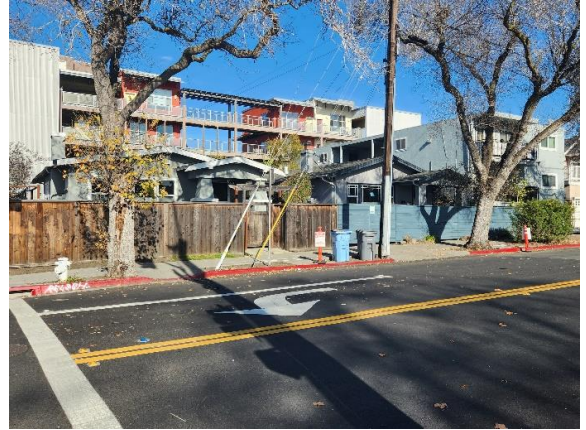
Figure 15: Single-family and multi-family residential buildings north of subject building at 1101 through 1109 Parker Street, with multi-family residential building in background at 2577 San Pablo Avenue. Looking north.
