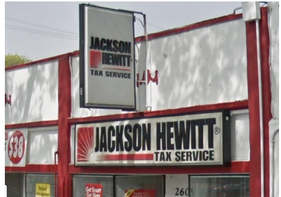
Figure 17: 2603-2605 San Pablo Avenue, April 2011. Note one of the mounting poles from the upper sign penetrates the center of the cartouche, which has been removed in this picture and replaced with red paint within its former silhouette. Source: Google Streetview.
