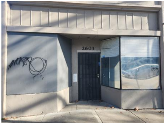
Figure 2: Detail view of north storefront on west façade. Looking east.
