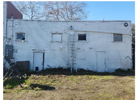
Figure 7: View of east façade. Looking west.
