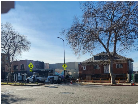
Figure 10: One and two-story commercial buildings south of subject building at 2634 through 2622 San Pablo Avenue. Looking southwest.
