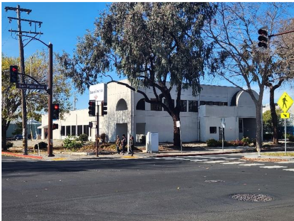
Figure 16: Two-story commercial building northwest of subject building at 2546 San Pablo Avenue. Looking northwest.
