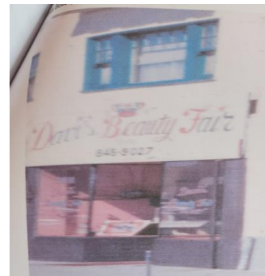
Figure 19: 2611 San Pablo Avenue storefront, circa 1970. Note divided lites in the second story windows and tile bulkhead, not extant. Image bent at upper left corner. Source: Berkeley Architectural Heritage Association.
