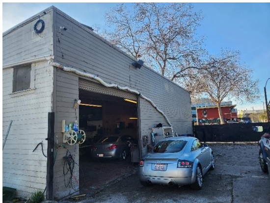
Figure 6: Oblique view of north facade. Looking southwest.
