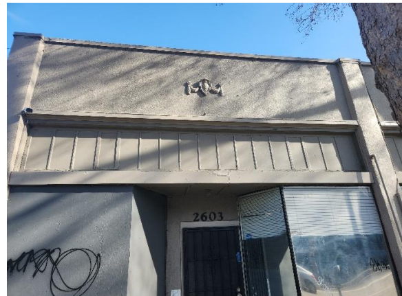
Figure 3: Oblique view of north half of west façade. Looking east.
