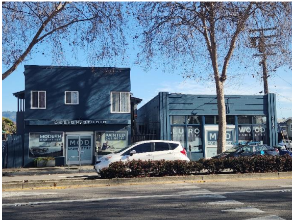
Figure 10: One and two-story commercial buildings south of subject building at 2617 and 2619 San Pablo Avenue. Looking east.
