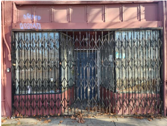
Figure 4: Detail view of south storefront on west façade. Looking east.
