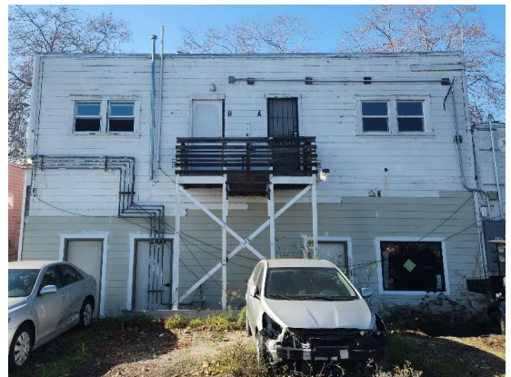
Figure 7: View of east façade. Looking west.
