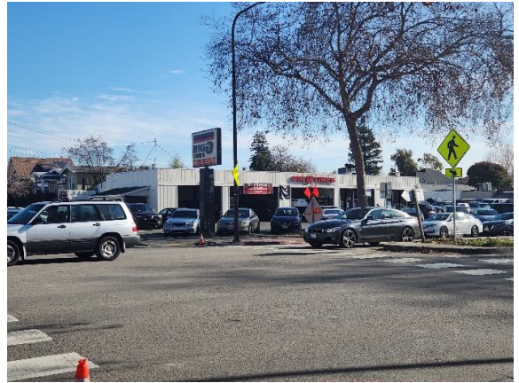
Figure 9: One-story commercial building south of subject building at 2625 San Pablo Avenue. Looking east.
