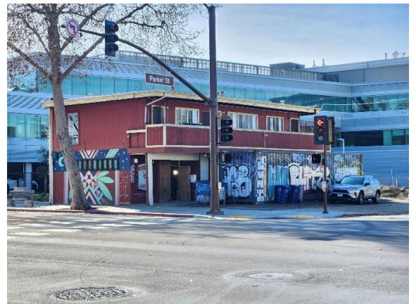
Figure 13: Two-story commercial building west of subject building at 2600 San Pablo Avenue. Looking southwest.
