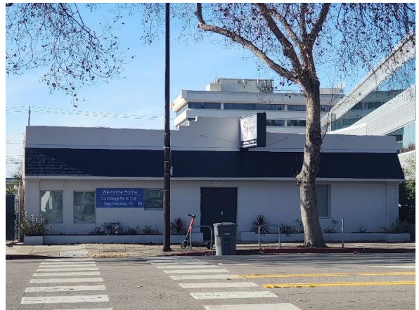
Figure 11: One-story church south of subject building at 2618 San Pablo. Looking west.
