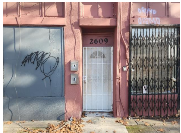
Figure 3: Detail view of the entrance to the 2609 San Pablo Avenue apartments, at the center of the west façade. Looking east.
